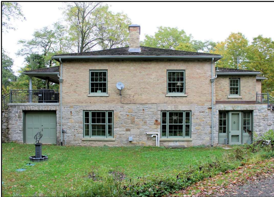
15. The south elevation of Park Farm cottage from the top of the laneway. The walk-out level lower level or basement was added in the c. 1930.
