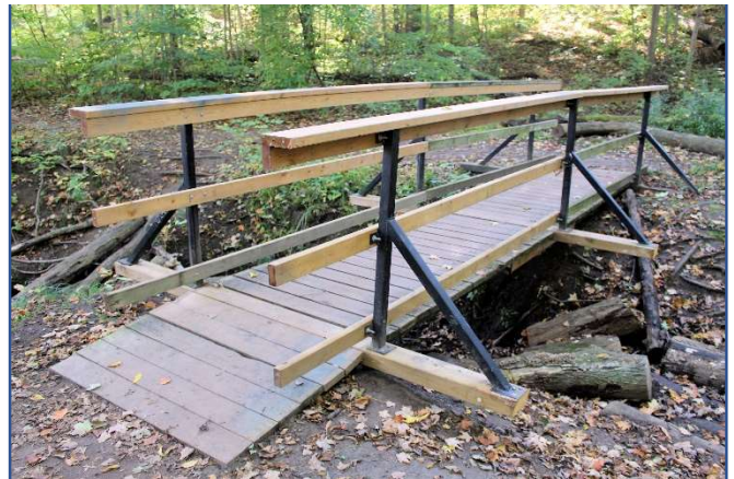
43. Walking trail bridge in Meadowlily Woods ESA.
