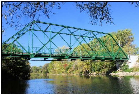
East elevation (view looking westward)
