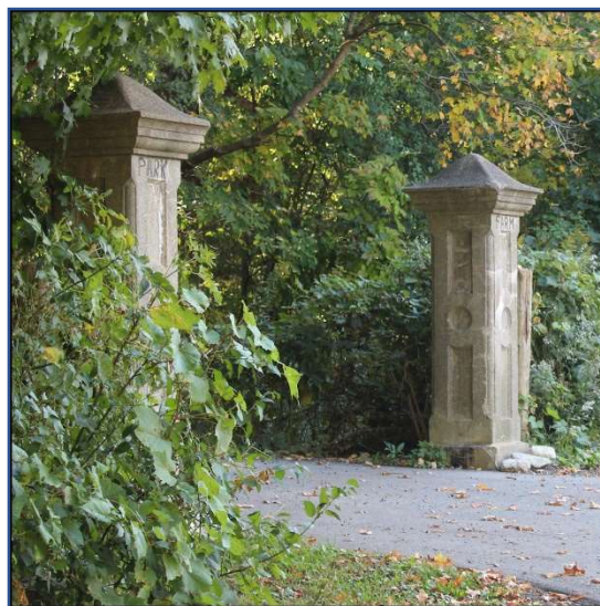
20. Cast masonry gate posts, likely from the beginning of the 20 th century, mark the ascent up to Park Farm cottage.
