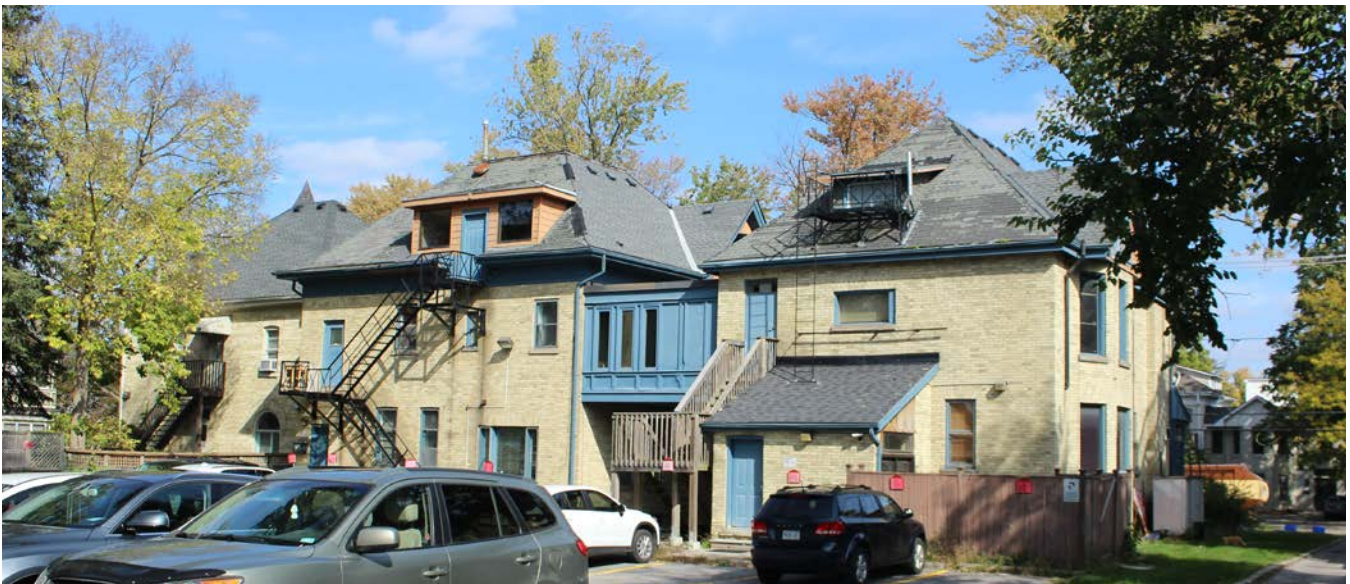
Image 7: 551-555 Waterloo Street: West/Rear Elevation with parking area. A contemporary dormer with an access door has been added to the upper half storey at the rear of 555 Waterloo Street, and a small addition added to the ground floor of 551 Waterloo Street at grade. The pedway can be seen connecting the two properties at second storey with a pathway below. Contemporary additions and exit staircases have also been added to the rear. Google Streetview, 2020.
