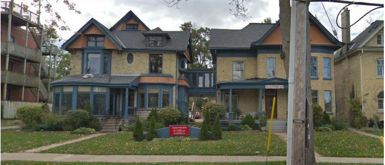
Image 6: 551-555 Waterloo Street: East/Front Elevation. Note two and a half storey massing, decorative gables, woodwork and projecting bay/window forms and window details. These aspects are significant within the HCD as they contribute to the visual consistency of the district as identified in the architectural character elements within the designation under Part V (OHA). Some original features appear to remain, while many have been replaced. The two properties have been modified with the addition of a contemporary pedway at the second storey (rear). The overall heritage value lies in its location and grouping, and remaining architectural merit as Victorian style residences, contributing to the overall context of the value of the HCD. Google Streetview, 2020.
