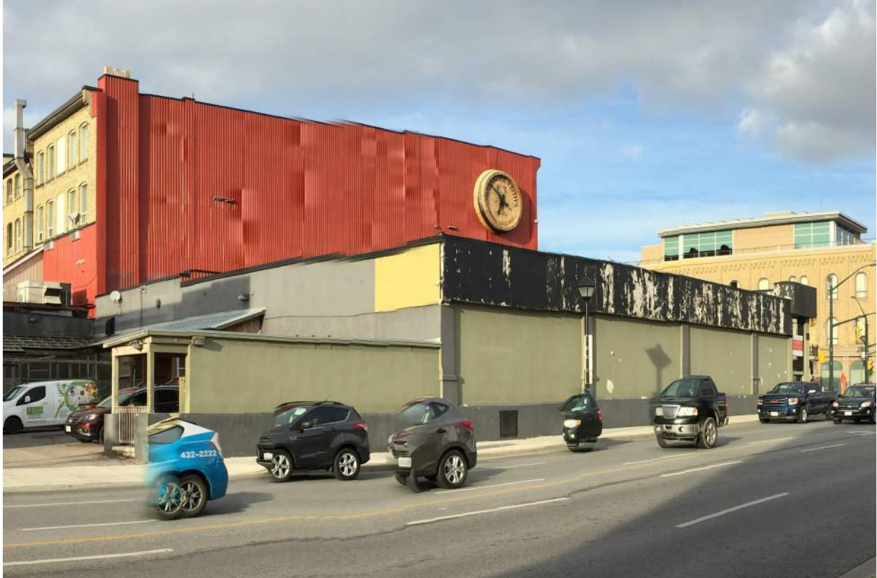
329 Richmond Street - Current Condition View of Existing South Elevation from Southwest
