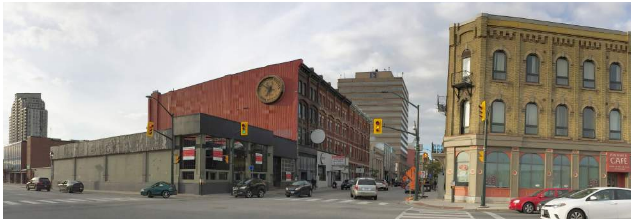
Current Site Photo - View looking northwest from York Street
