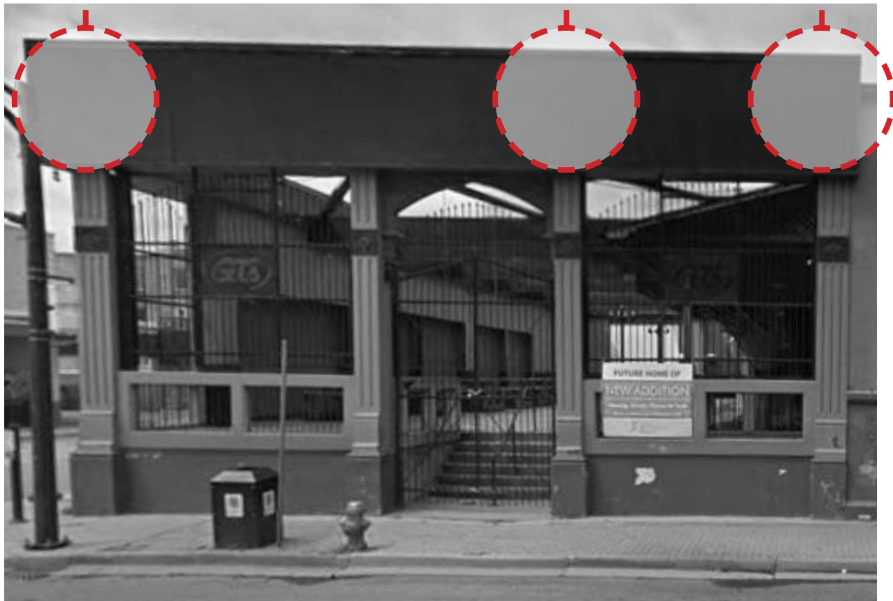
329 Richmond Street - Current Condition East Elevation
