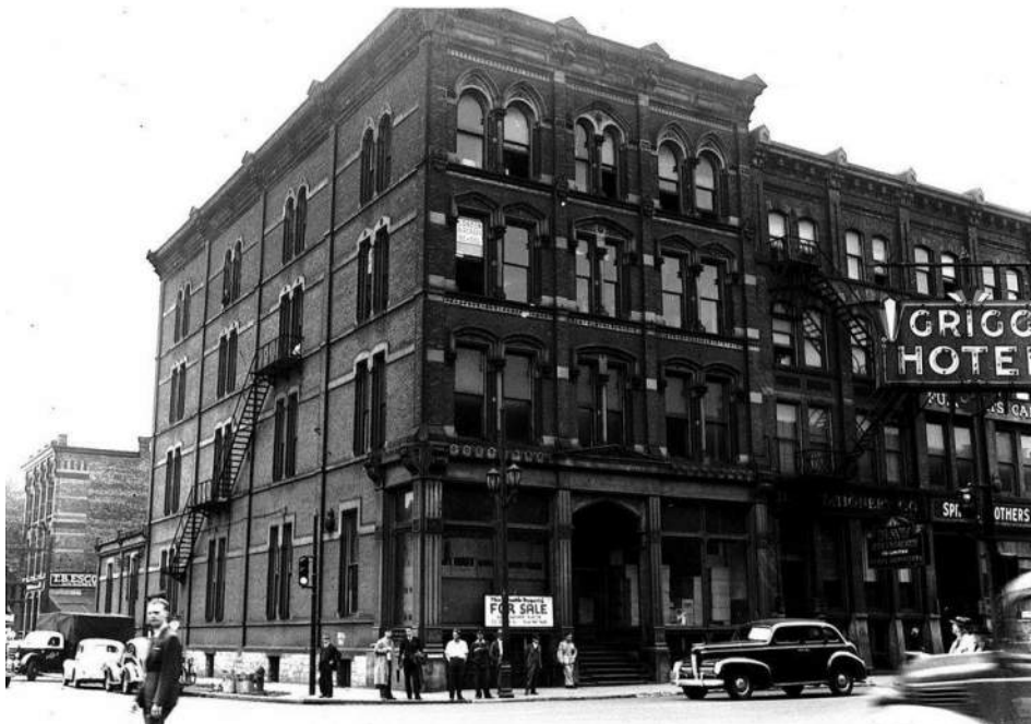
*View of 329 & 331 Richmond Street from East
