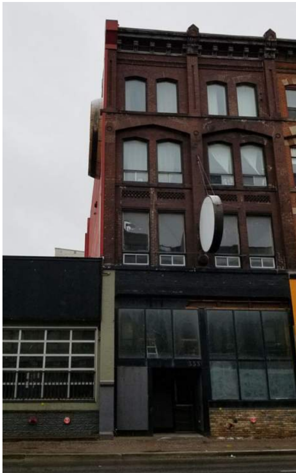
333 Richmond Street - 2018 East Elevation, Pre Construction
