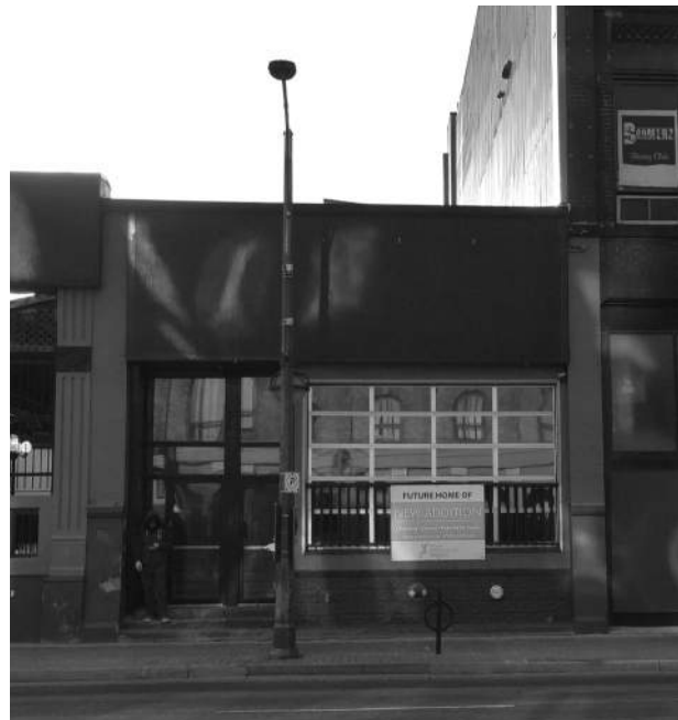
2016 - 331 Richmond Street, East Elevation
