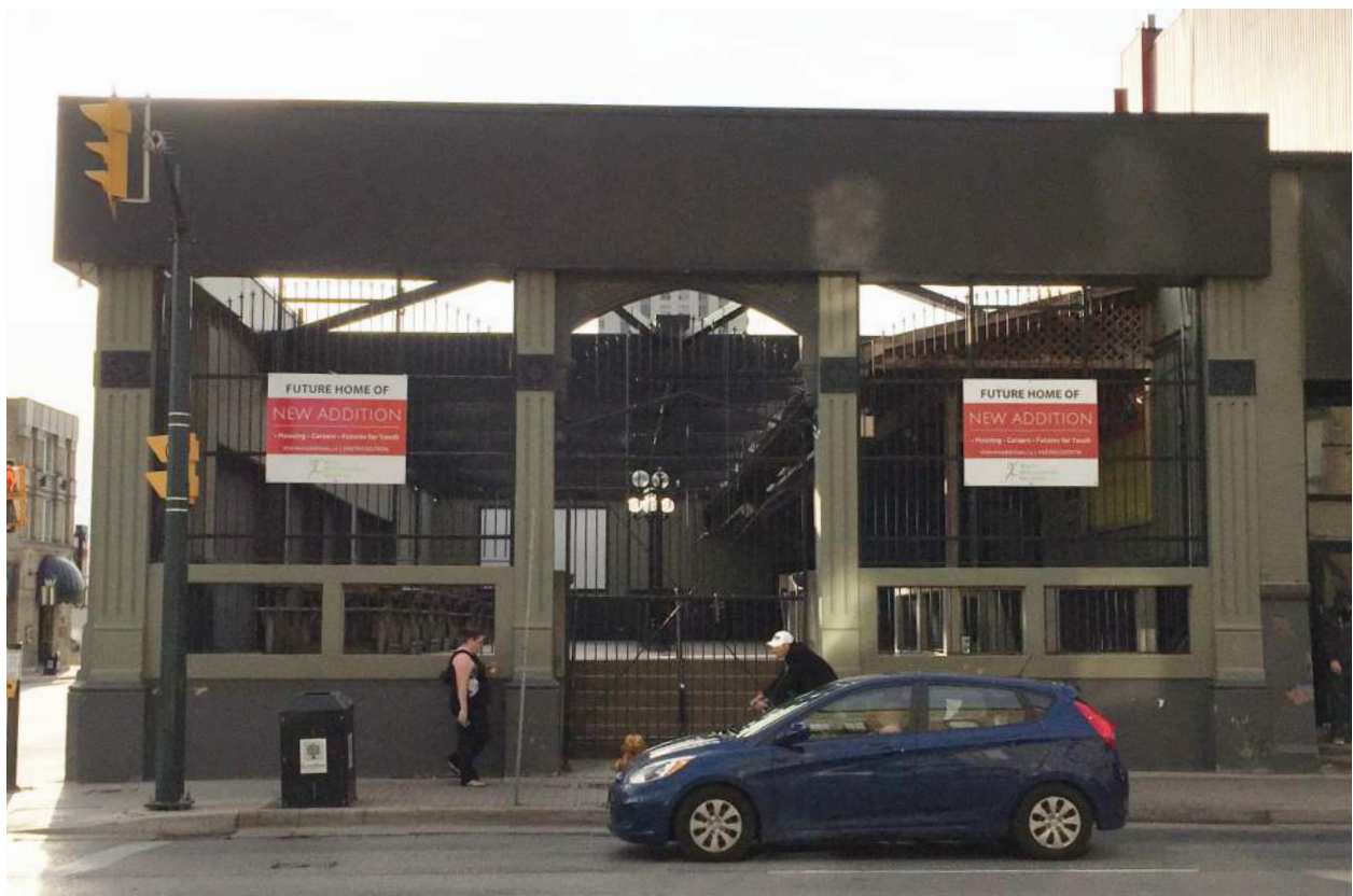
329 Richmond Street - Current Condition East Elevation
