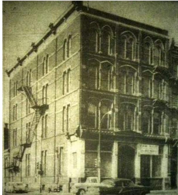
*View of 329 Richmond Street from East
