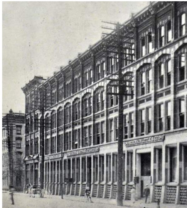
*View from Richmond Street Looking Southwest
