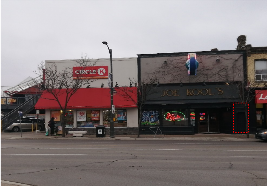
Figure 40 —View of front façade of 595 Richmond Street including restaurant “Joe Kool’s” to the north and “Circle K” to the south; red box indicates location of access between 595 and 599 Richmond Street to rear ancillary brick structure (Source: MHBC, 2020)
