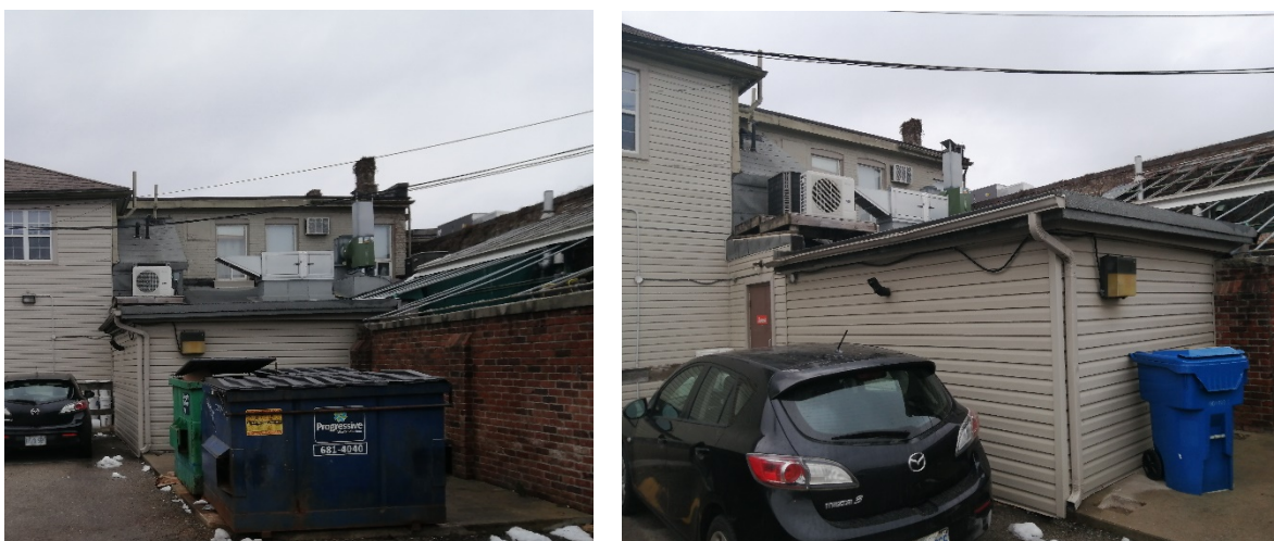
Figures 26 & 27 – (left) View of west elevation (right) View of west elevation looking south-east (Source: MHBC, 2020)
