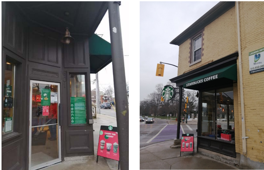
Figures 34 & 35 – (left) View of entrance to 601 Richmond Street via south-west corner of the intersection at Richmond Street and Central Avenue. (right) View of front façade looking south, (right) View of entrance at corner of the intersection looking south-east (Source: MHBC, 2020).
