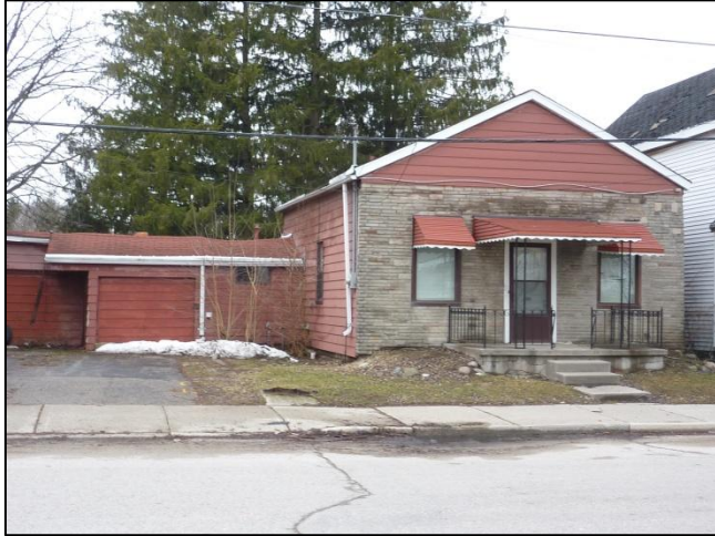
275 Thames –former chapel (Priority 1) (attached garage – later addition)
