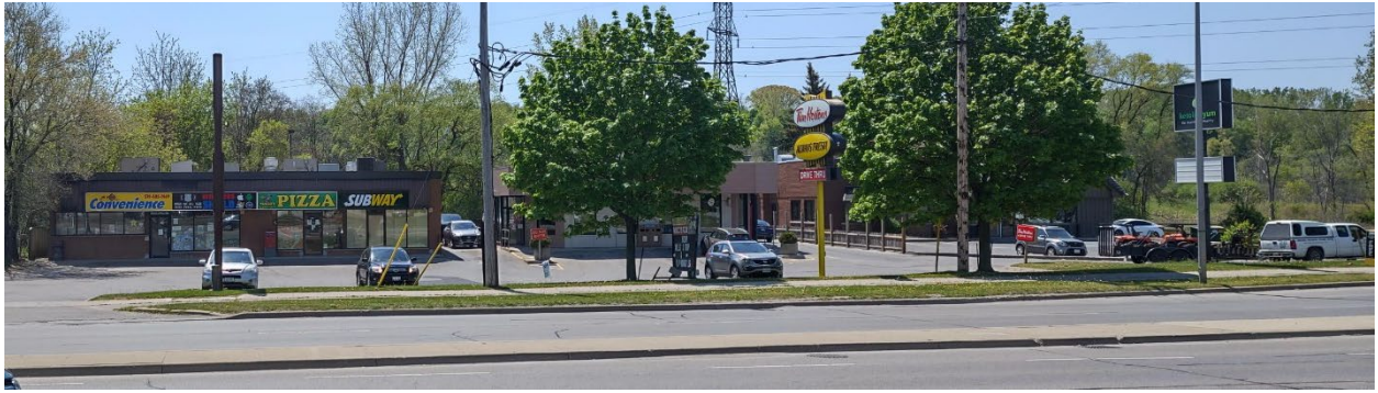
Figure 1: 915-919 Commissioners Road East Plaza
