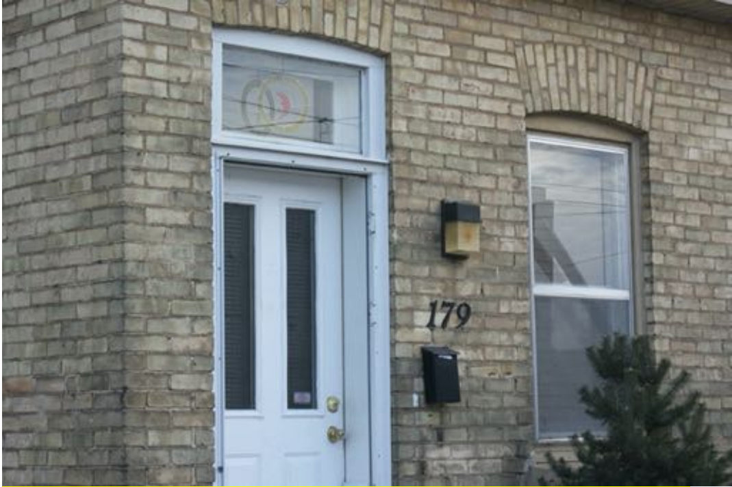
Closeup of front doorway of 179 Ann Street, showing voussoir in detail.
