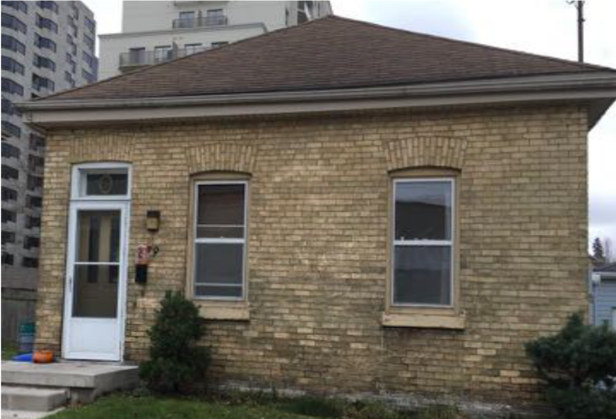
Front of 197 Ann Street, illustrating original voussoirs above door and the two front windows. (Photo Credit: Hayley Caldwell).
