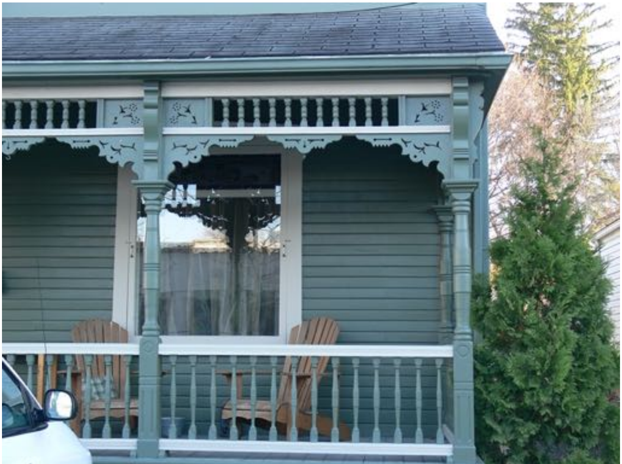
127 Ann Street, home to James Arscott, originally of the Arscott Tannery which was almost immediately to the east of 127 Ann Street. James Arscott was later foreman of the Hyman Tannery.
