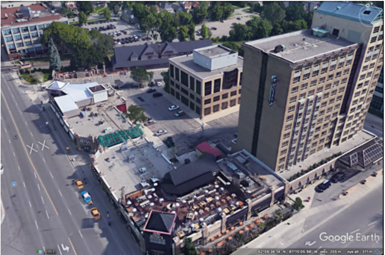
The Station Park development added density while incorporating the 1892/93 CPR railway station.
