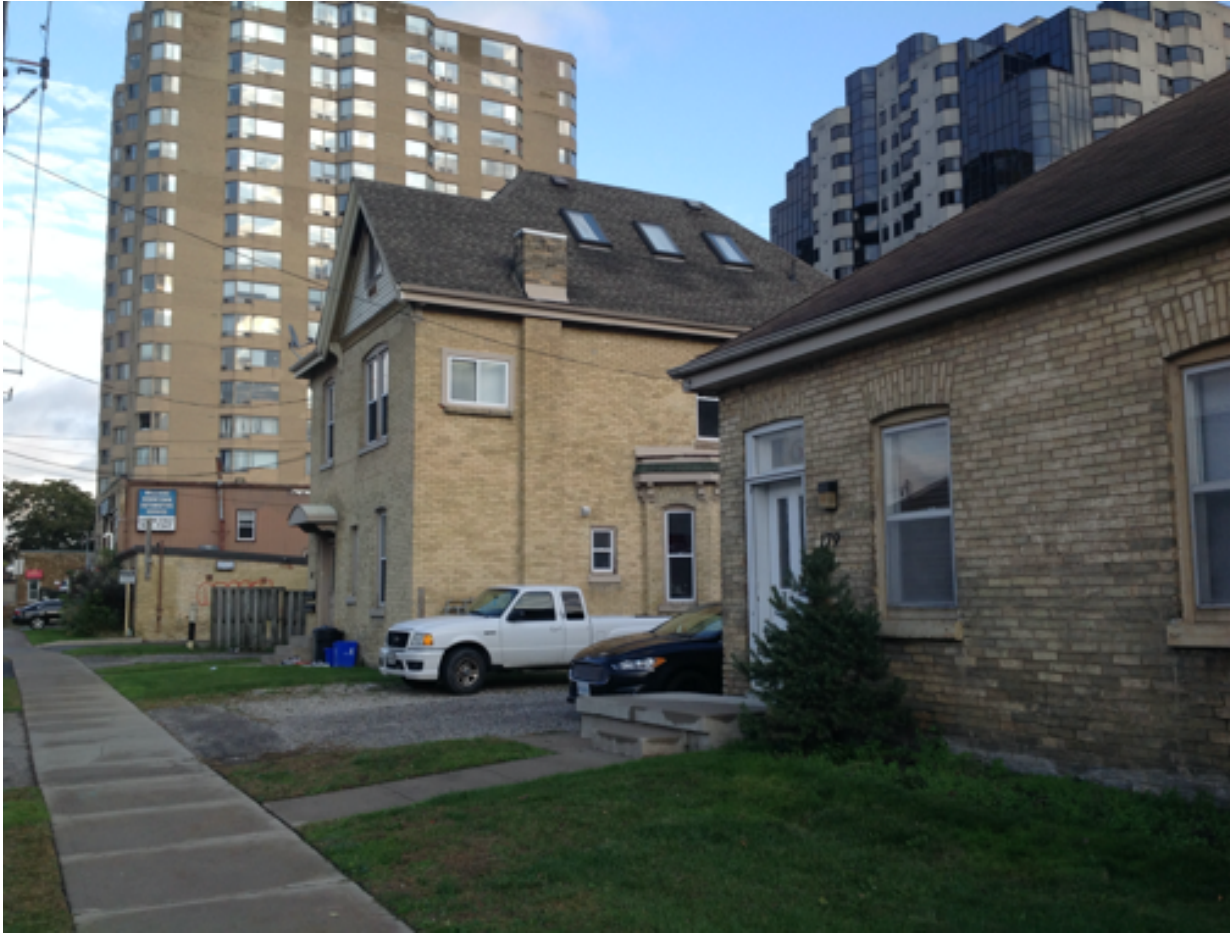
The Kent brewery (far left) and the two residences associated with it, 183 Ann Street (centre) and 179 Ann Street (right), illustrating Kent Brewery site looking east. The brick on 183 and 197 echoes the brick on the cottage at 179. John Hamilton owned all of these properties, and Joseph Hamilton lived in both 183 and 179 Ann Street at different times. The only other identifiable example in Canada of an extant brewery building with the brewer's house still intact next door is Alexander Keith's brewery in Halifax (see Appendix D)
