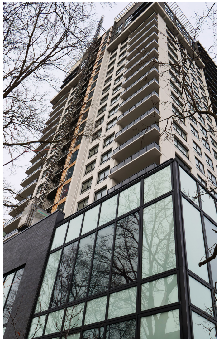
This image shows a podium at a human-scale with the building height and bulk set back from the street edge.
