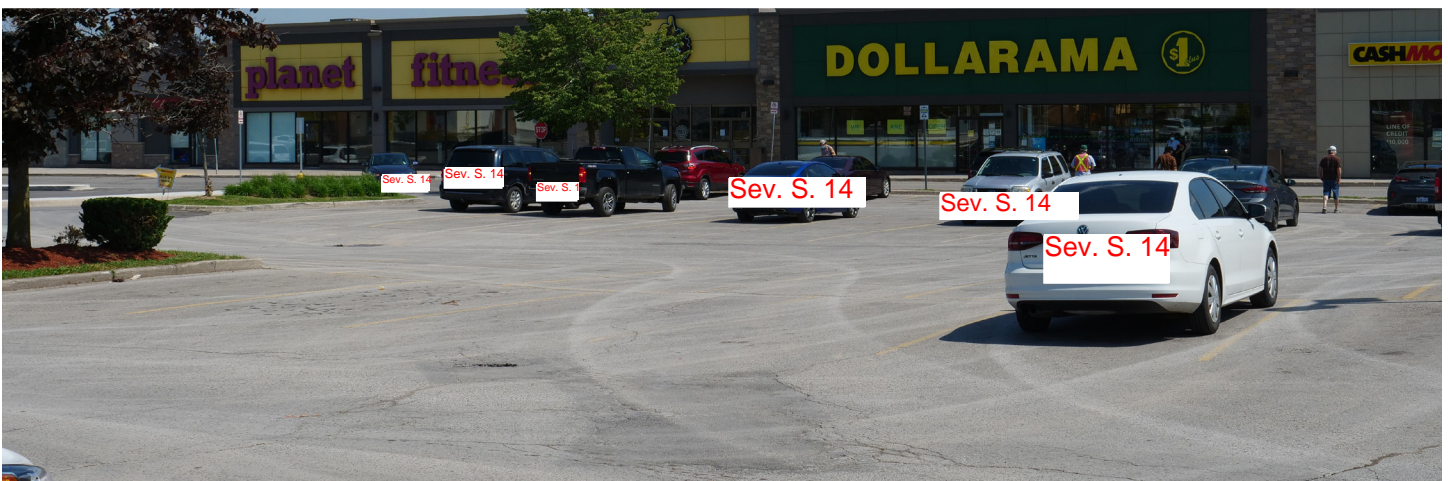
This image shows a development with large amounts of surface parking at the front of the site.
