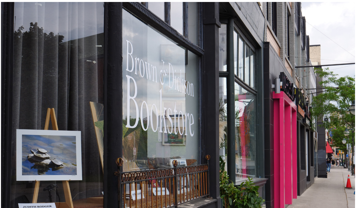
An example of a street with active ground floor activities in London.
