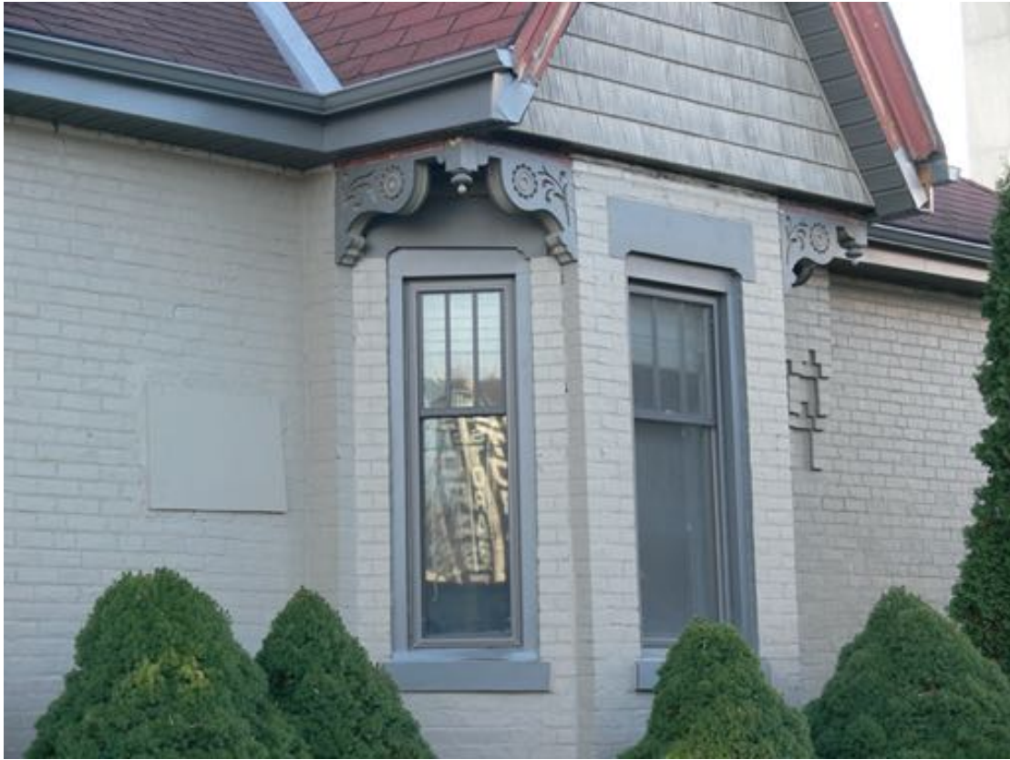
724 Talbot Street (home to Edward Boles, labourer and later foreman of Carling's Brewery). Note the bay window with a Talbot North lintel, similar to 197 Ann Street.
