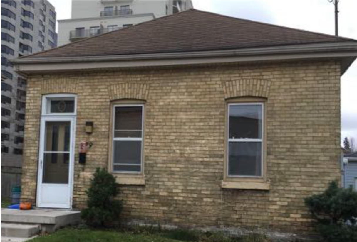
Front of 197 Ann Street, illustrating original voussoirs above door and the two front windows. (Photo Credit: Hayley Caldwell).
