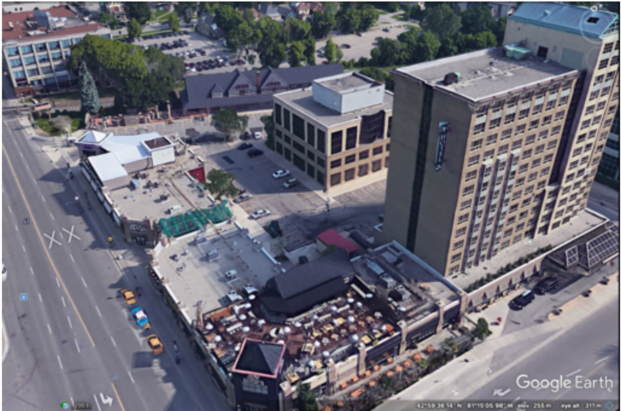
The Station Park development added density while incorporating the 1892/93 CPR railway station.
