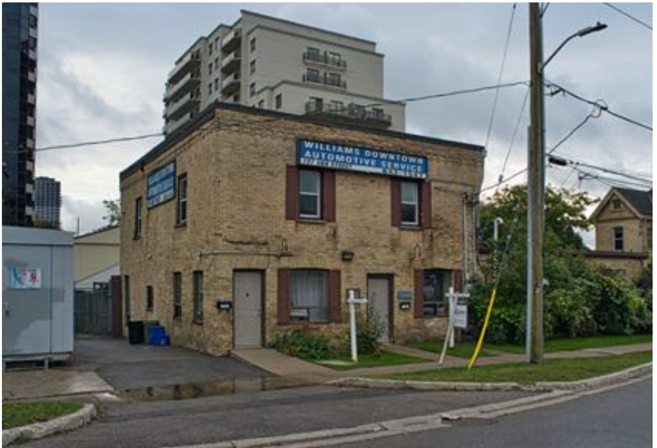
Kent Brewery building, October 2020
