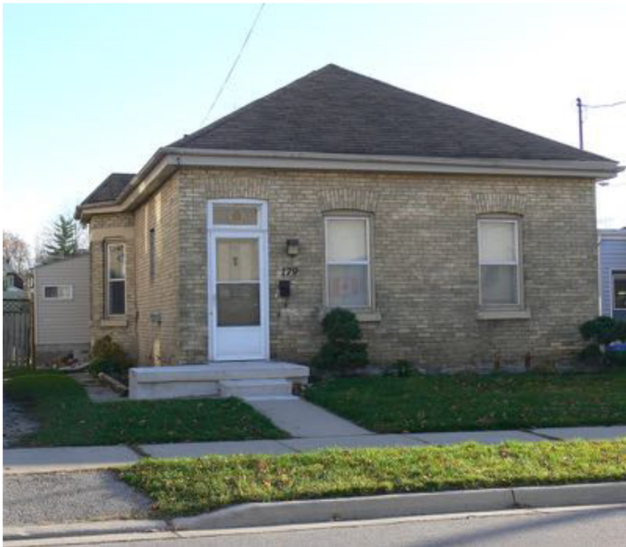
Front of cottage at 197 Ann Street, showing profile of bay window on left.
