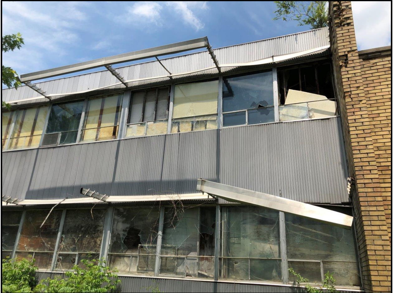
Photo 4 - front of abandoned building
