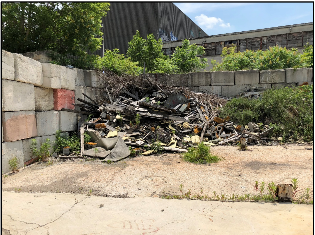
Photo 2 - rear of abandoned building
