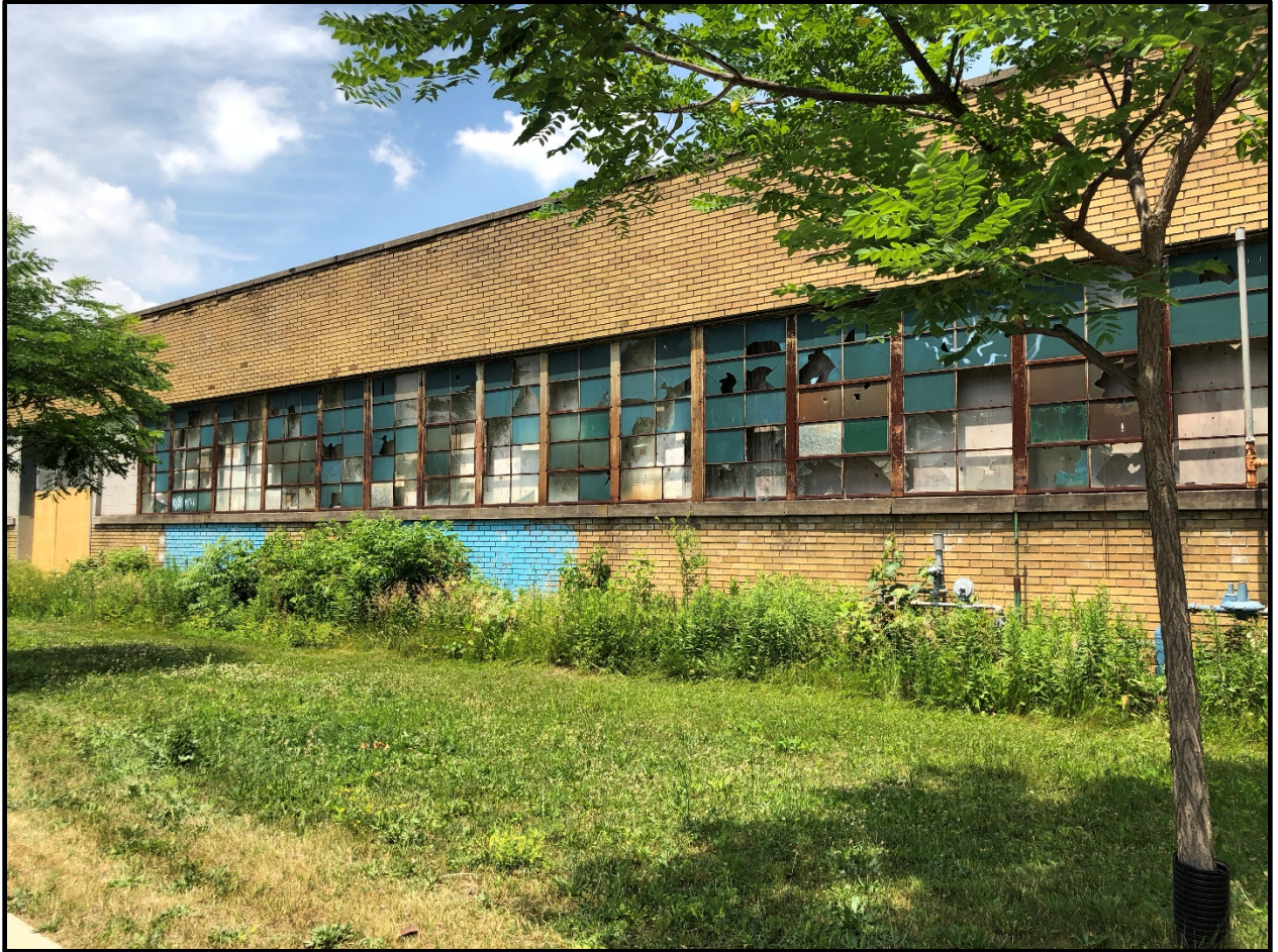
Photo 3 - front of abandoned building
