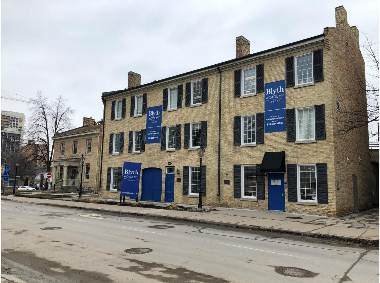
Figure 1: Existing buildings at 435 and 441 Ridout Street North
