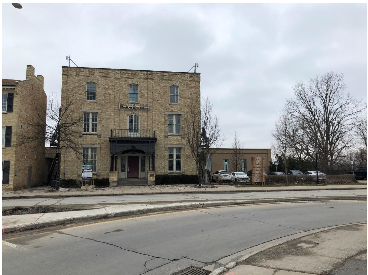
Figure 2: Existing building at 451 Ridout Street North
