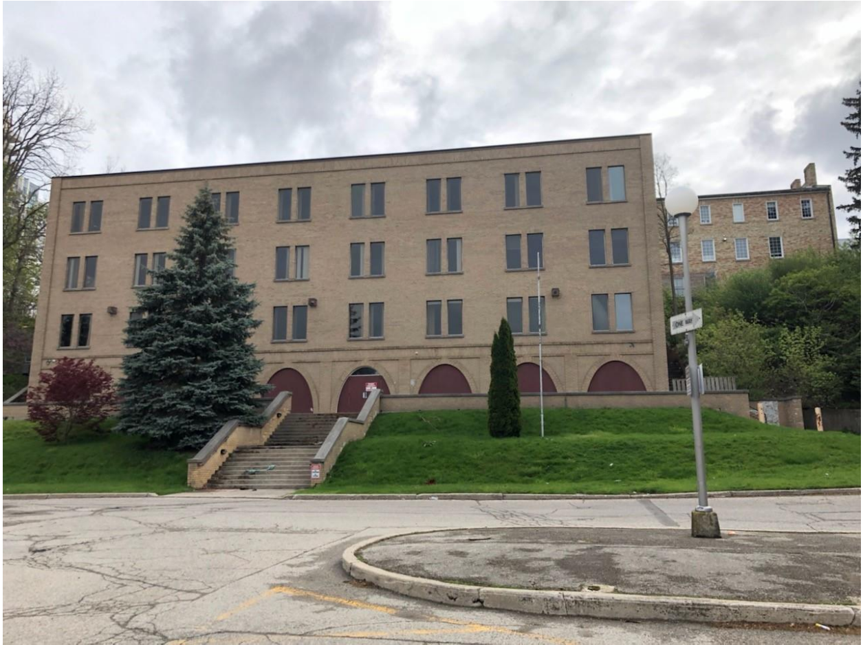
Figure 4: Existing building at 451 Ridout Street (view from lower parking area)
