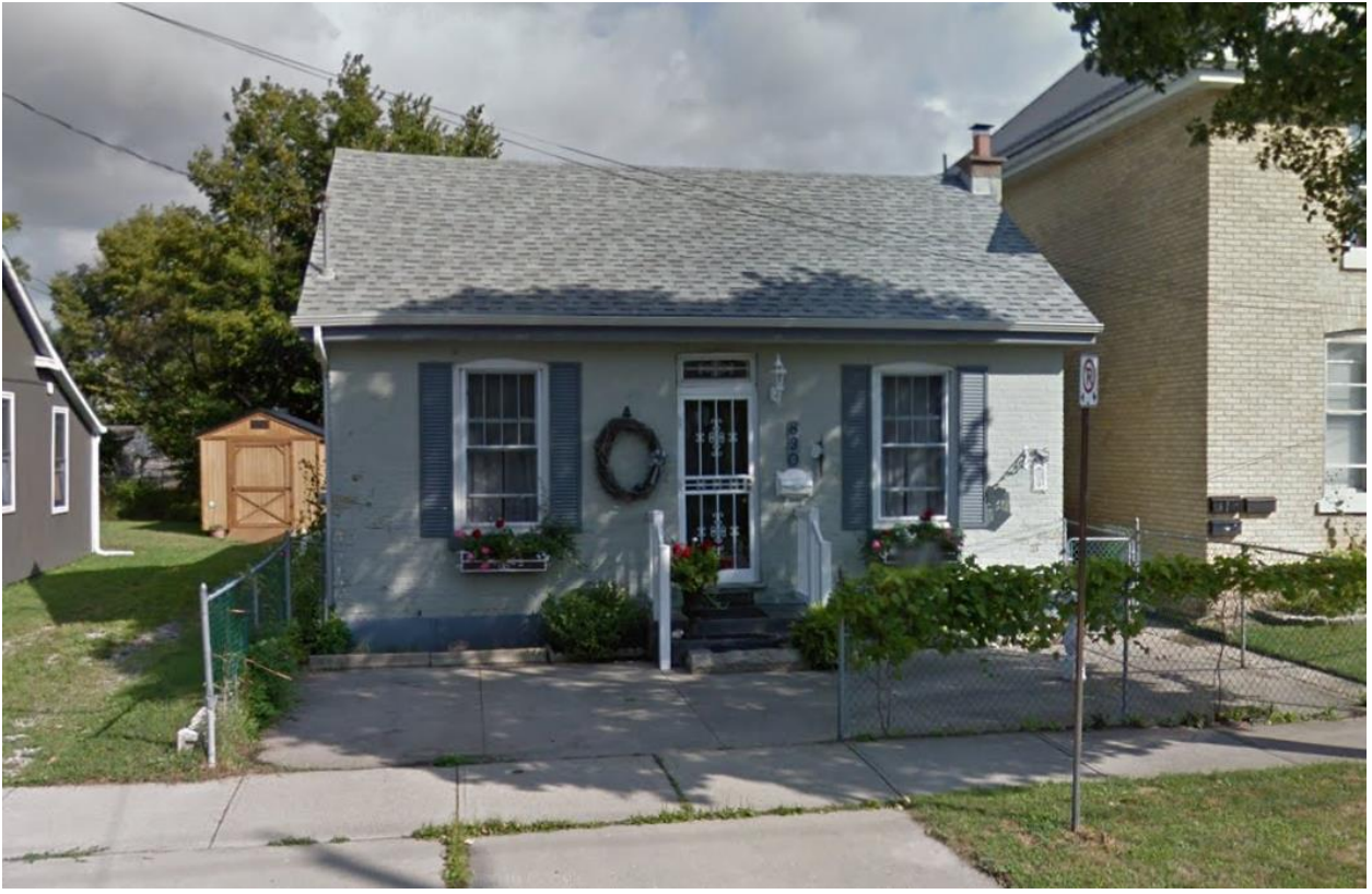
Image 22: Photograph showing the dwelling at 890 Trafalgar Street, a heritage listed property.
