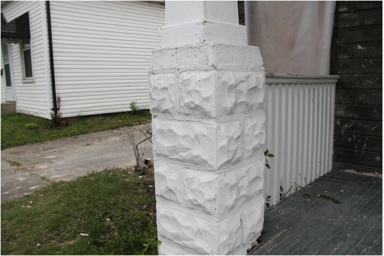
Image 9: Detail of the front porch material including rusticated concrete block, wood deck flooring, and wood rail and spindles, 2021.
