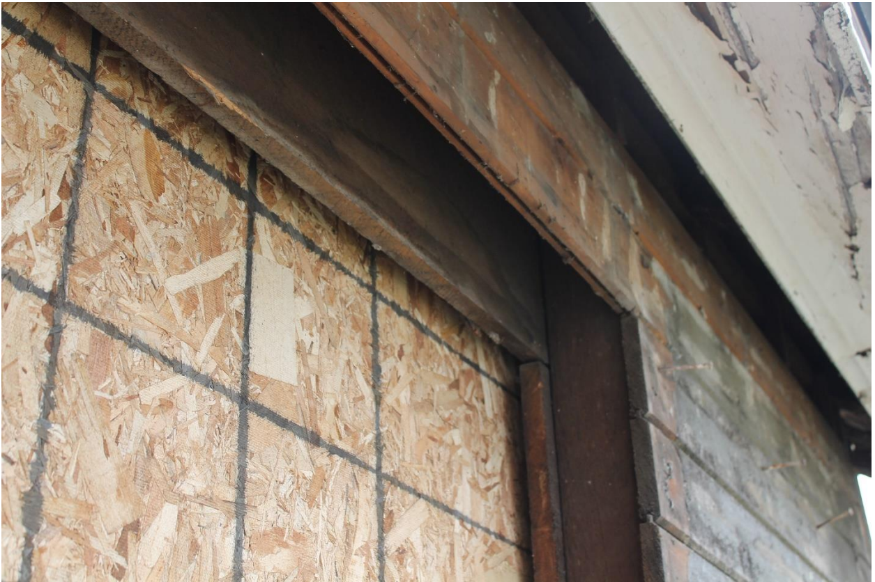
Image 10: Detail of window opening on the west (front) facade, showing details of tongue and groove siding, 2021.
