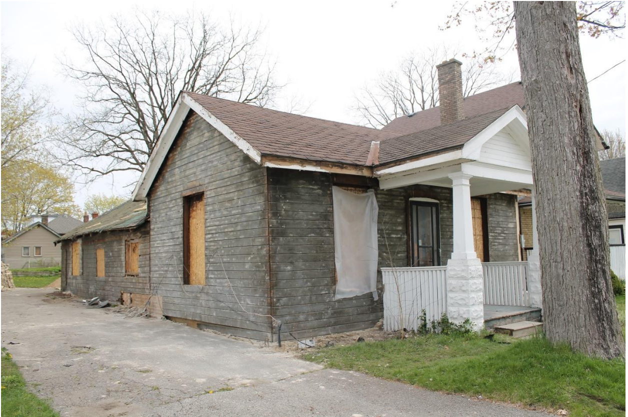
Image 7: Photograph showing the west (front) facade and north facade of the dwelling. The rear addition is visible, 2021.
