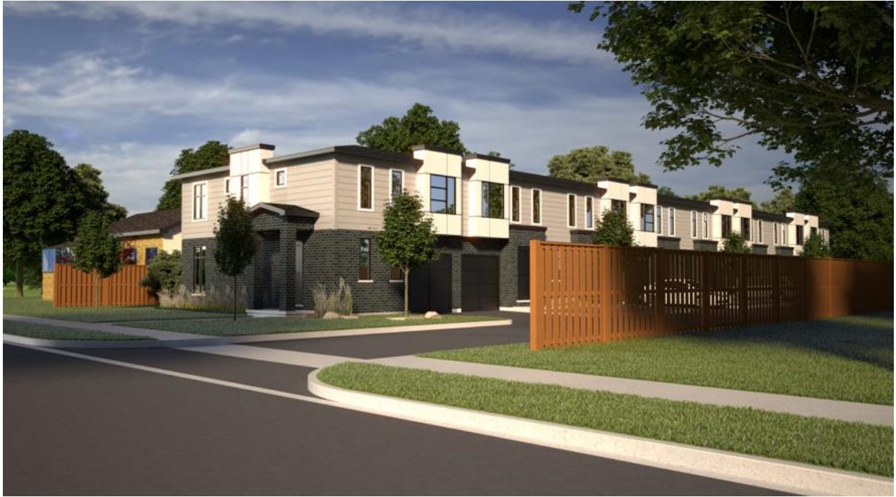
Figure 5 - Front view from Wethered Street looking northeast
