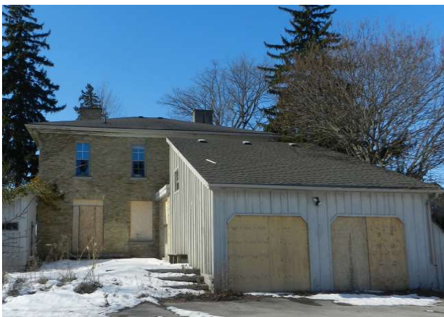
Image 3: East elevation. Photo: a+LiNK architecture inc.
