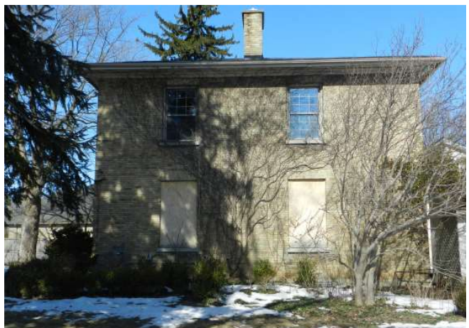
Image 4: South elevation. Photo: a+LiNK architecture inc.
