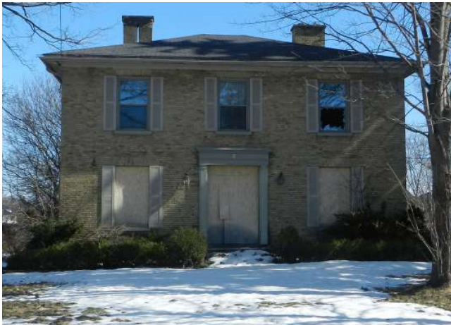
Image 1: Front façade (West elevation). Photo: a+LiNK architecture inc.
