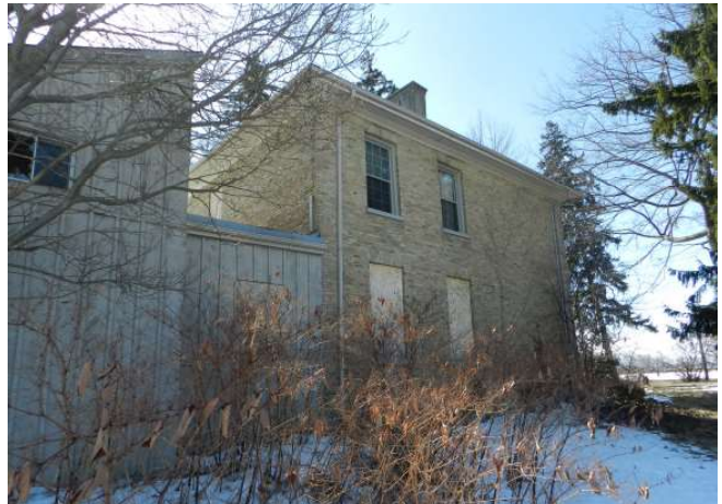
Image 2: North elevation. Photo: a+LiNK architecture inc.
