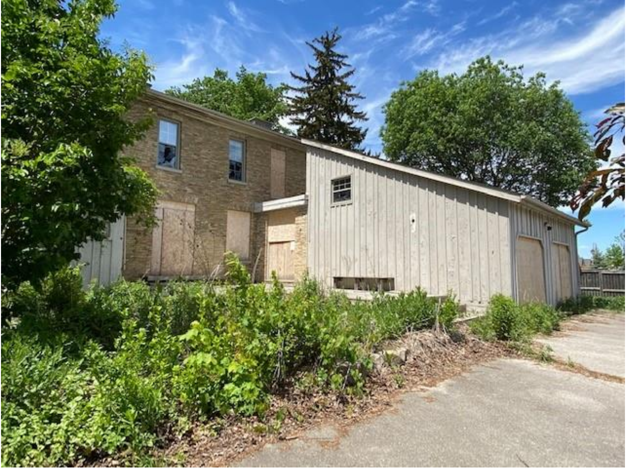
Image 4: View of rear elevation including contemporary addition (May 29, 2021)
