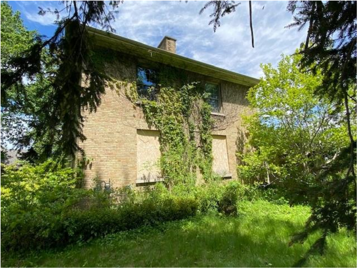
Image 3: View of south-side elevation (May 29, 2021)
