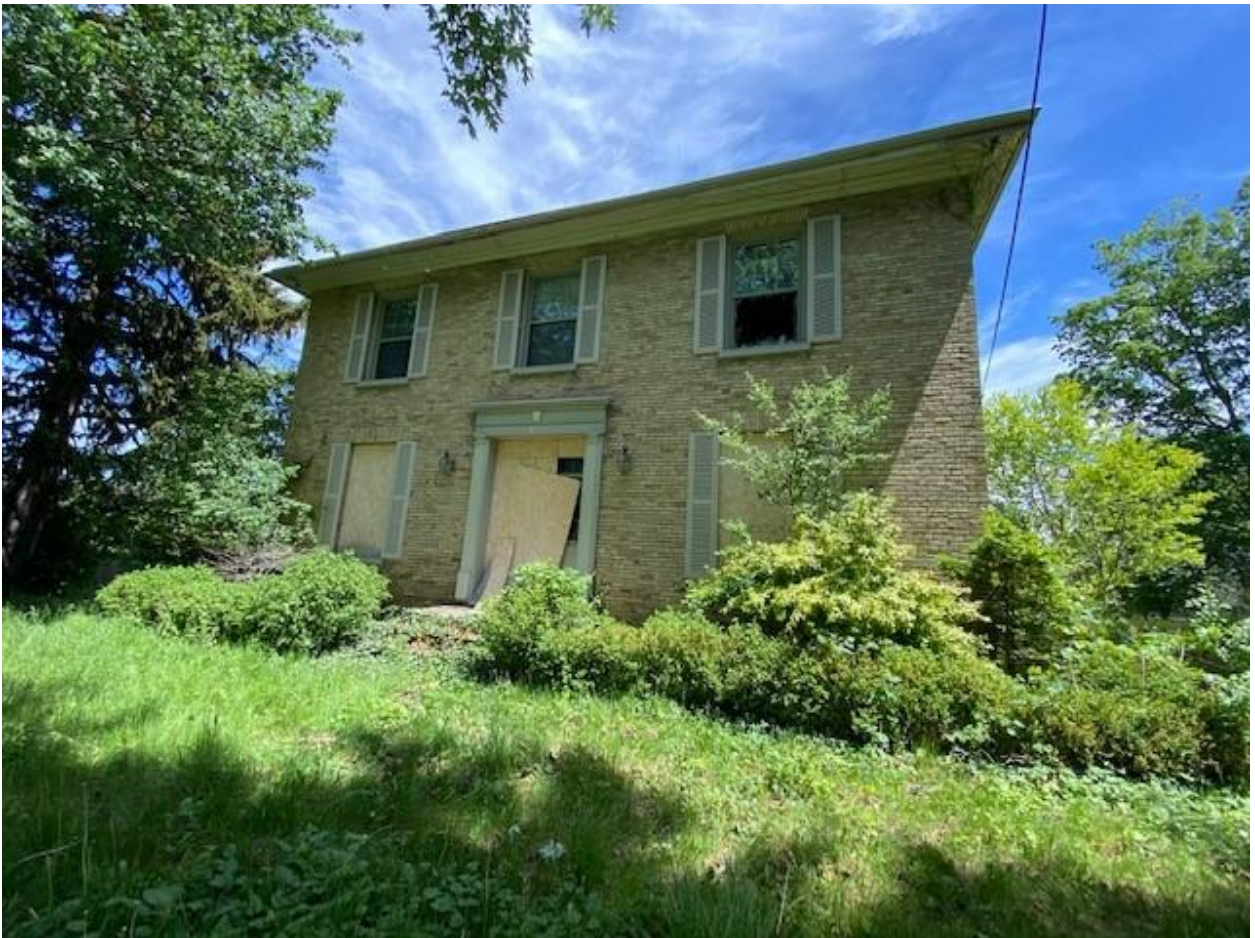
Image 2: Close-up view of façade (May 29, 2021)
