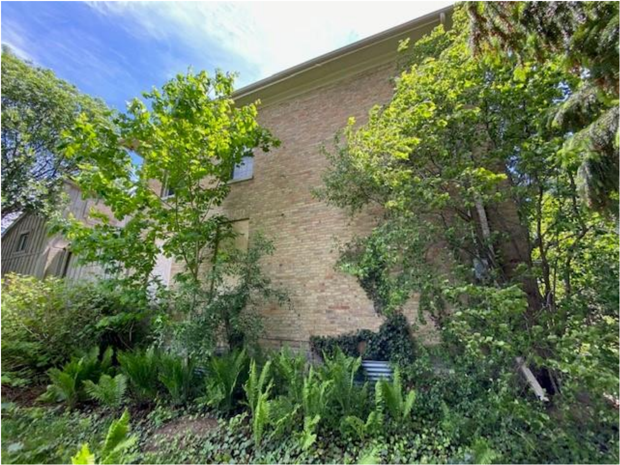
Image 5: View of north-side elevation, contemporary addition at rear (May 29, 2021)
