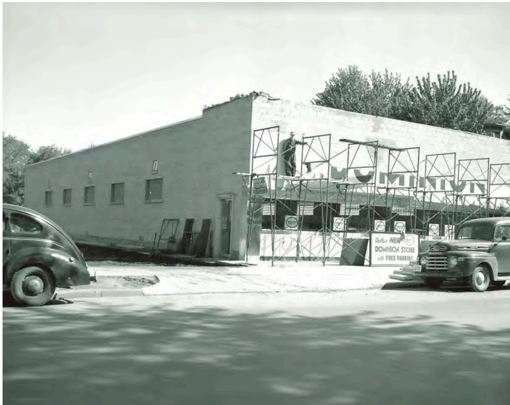
Figure 10: Photograph of the construction of the Dominion grocery store at 496 Dundas Street, City of London on May 13, 1949 (Courtesy of the Western Archives, LFP Negative Collection).
