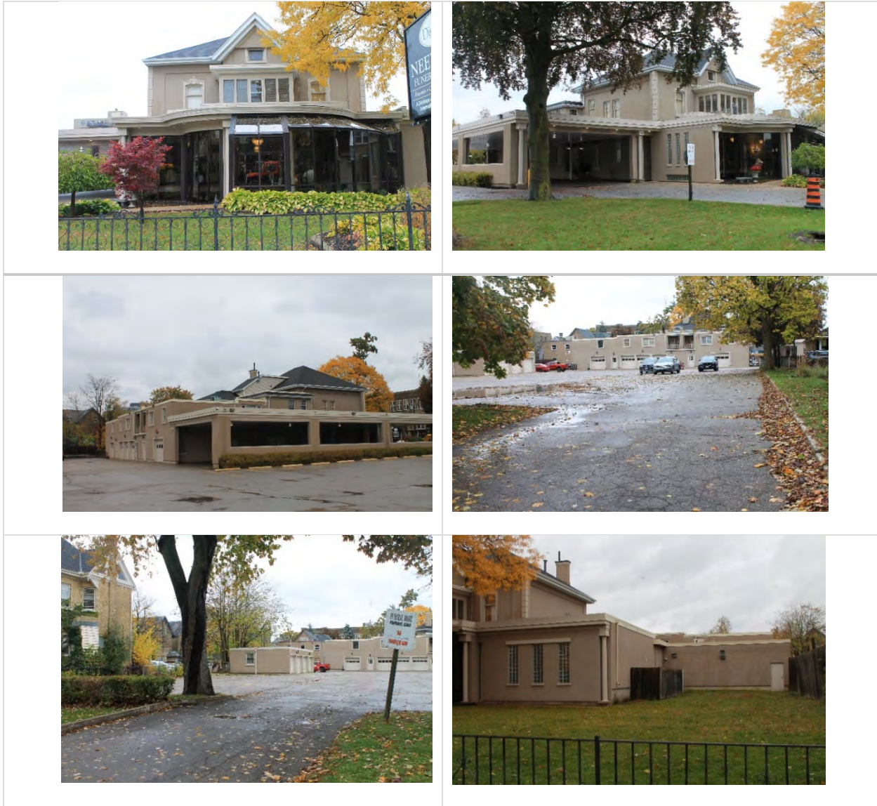
(Above left) Front elevation of building; (above right) West elevation of building; (middle left) West and north (rear) elevation of building; (middle right) Rear elevation of building; (below left) Rear elevation of the building; (below right) East elevation of building (Source: MHBC, 2020).
