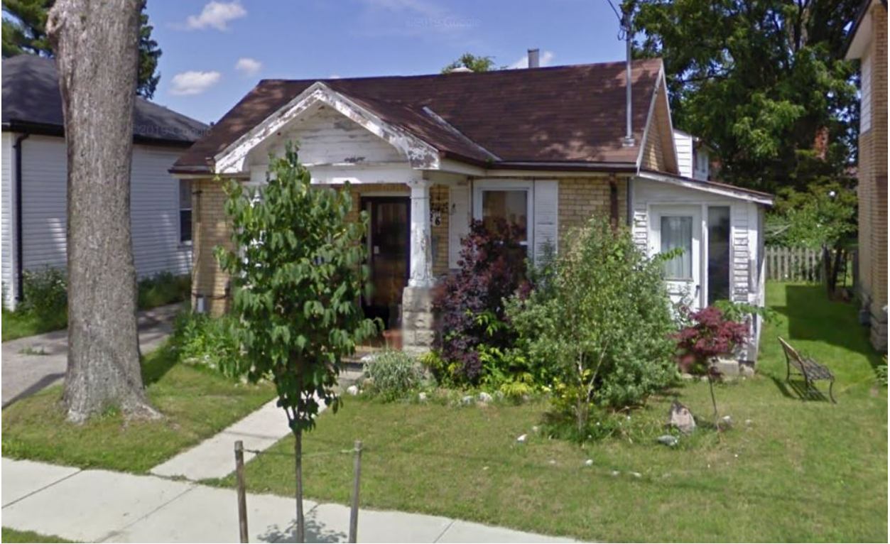
Image 1: Image showing the dwelling located at 126 Price Street, 2009 (Google Street).
