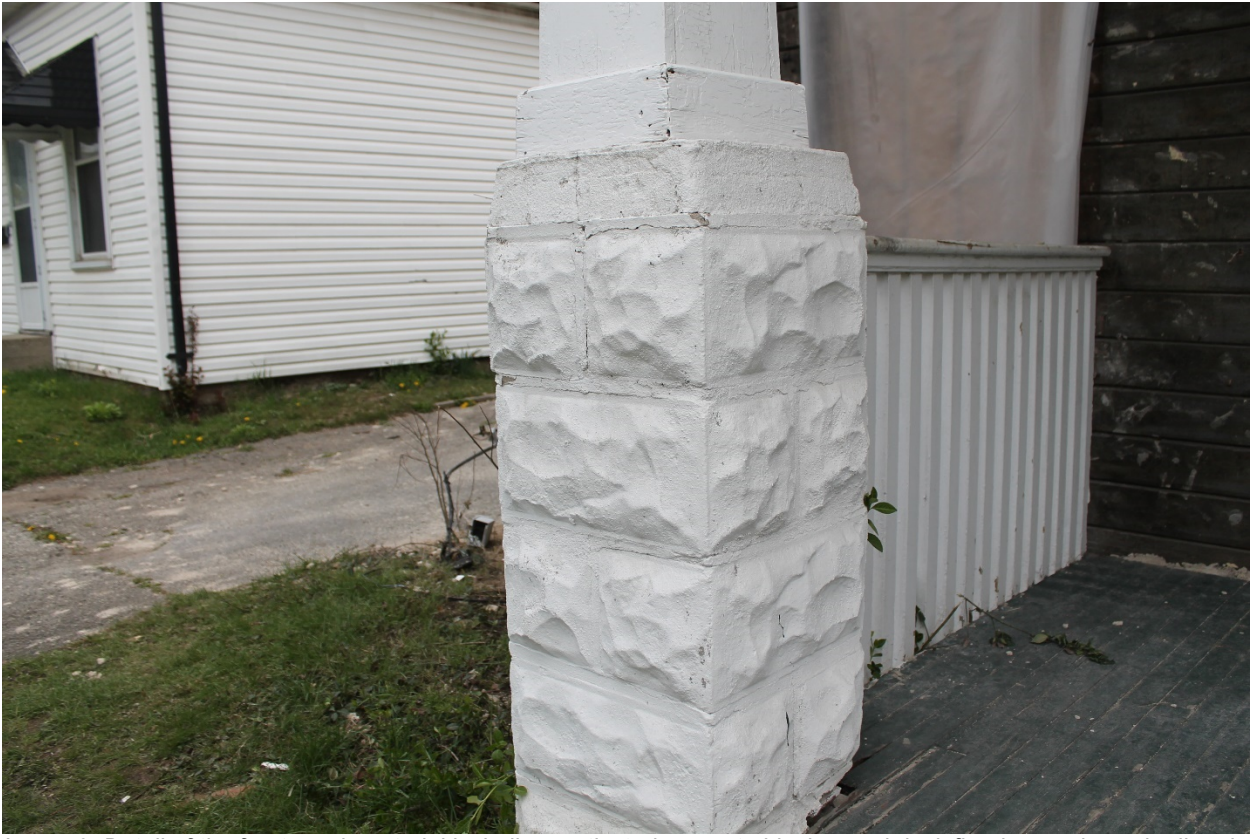
Image 9: Detail of the front porch material including rusticated concrete block, wood deck flooring, and wood rail and spindles, 2021.
