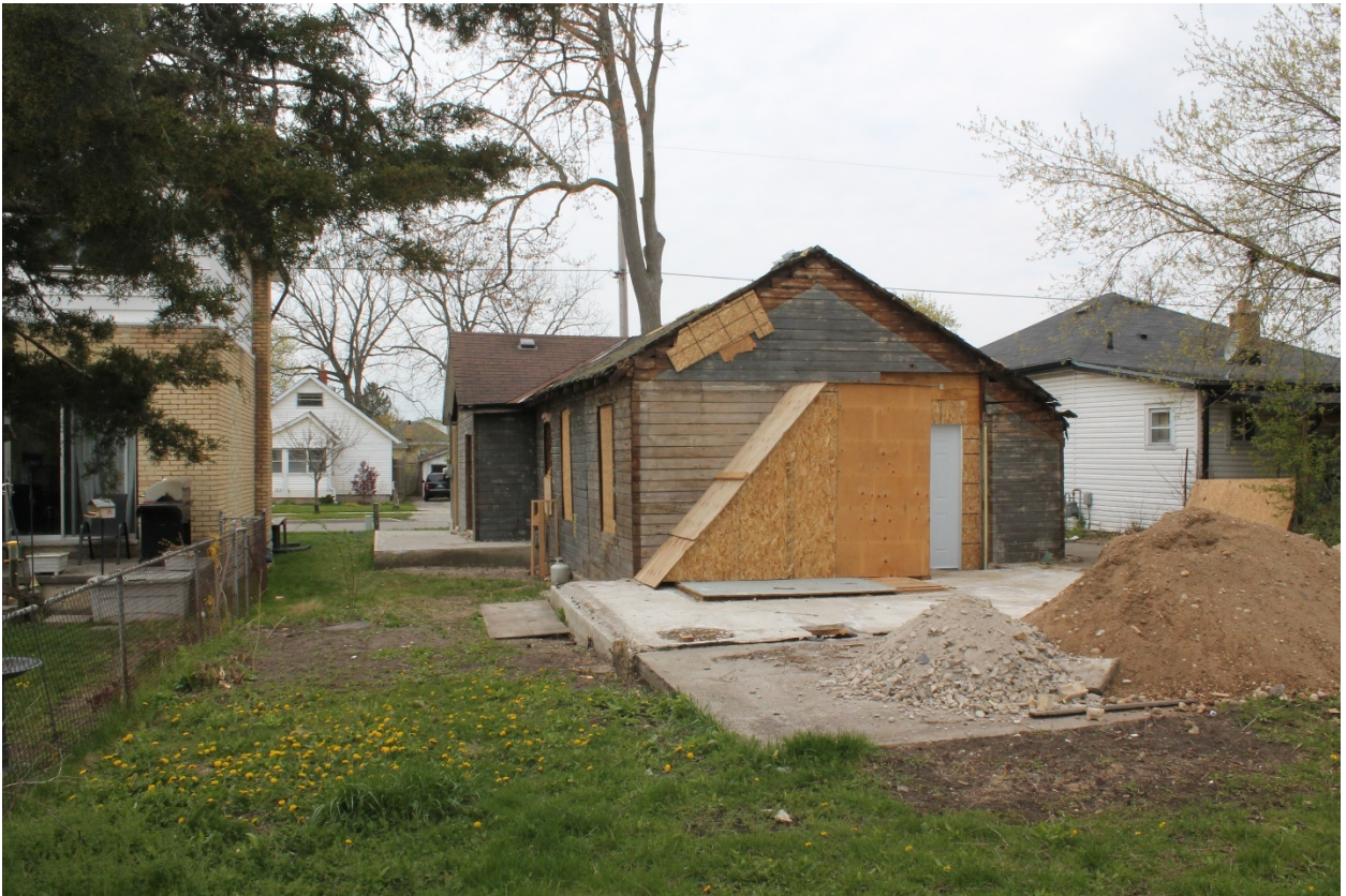
Image 12: Photograph looking east from the rear of the lot showing the back of the rear addition and footprint of the previously demolished two-storey addition, 2021.
