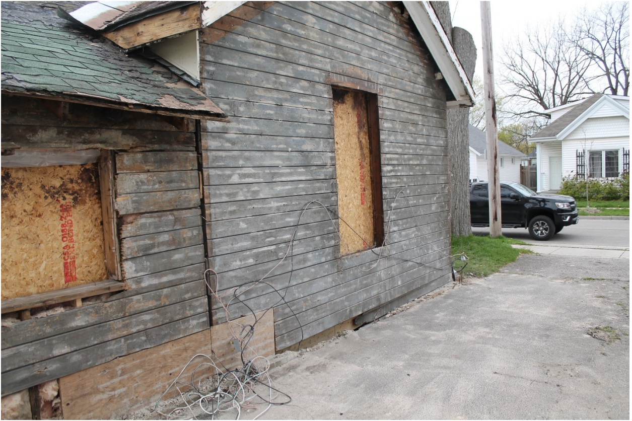
Image 11: Photograph looking east showing the intersection of the main dwelling (right) and the rear addition (left), 2021.
