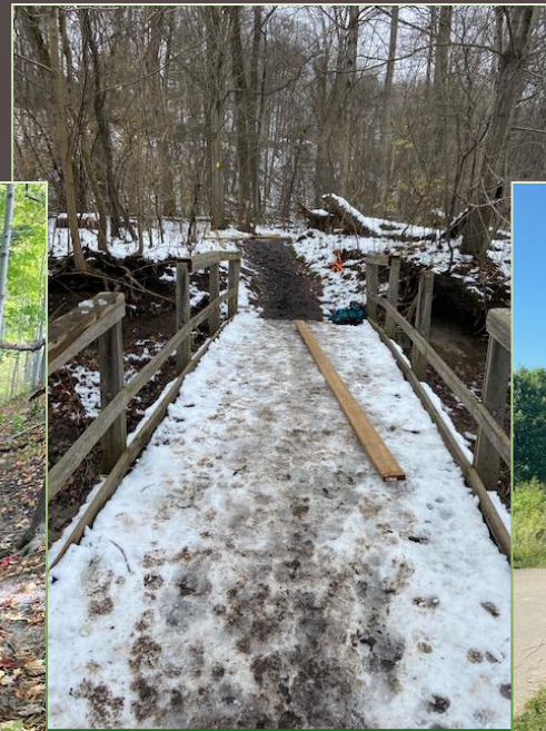
Metamora bridge railing repair
