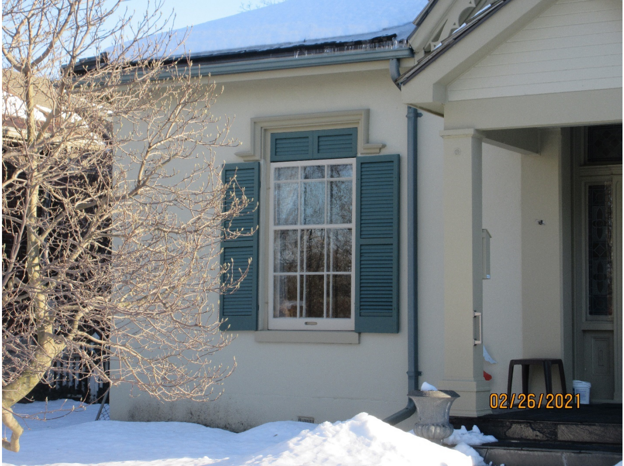
Image 16: View showing the easterly window, storm window, shutters, sill, and label on the front (north) façade of Carfrae Cottage.
