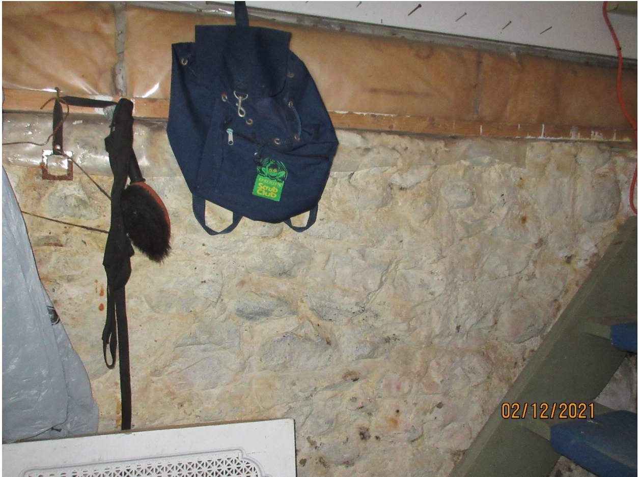
Image 7: Photograph showing an example of the rubble stone foundation construction of Carfrae Cottage, as seen in the basement.
