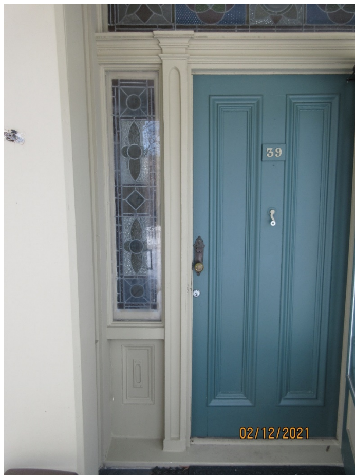
Image 12: Photograph showing the front doorway with single leaf, painted wood door with two long panels (which is believed to be original to the house), set in a rectangular opening with rectangular sidelights to both sides, a panelled dado below, and a rectangular transom. The sidelights and transom feature stained glass in repetitive geometric patterns with coloured and textured glass. The doorway is recessed in the façade with a plain reveal. The door opening is framed by pilasters with a Gothic point, with entablature supporting the architectural framework of the doorway.
