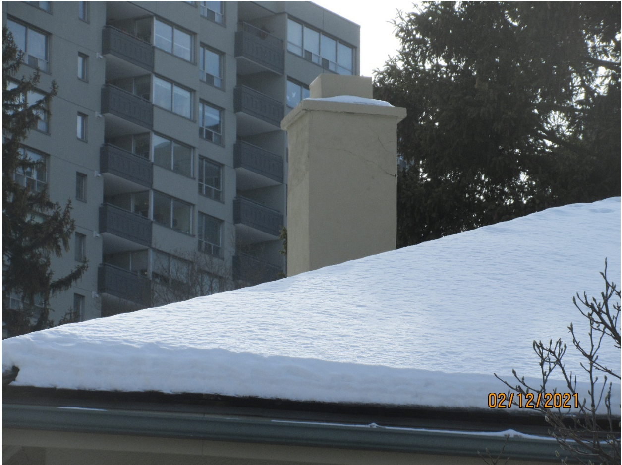
Image 9: Photograph of the east chimney, as seen from Carfrae Street.
