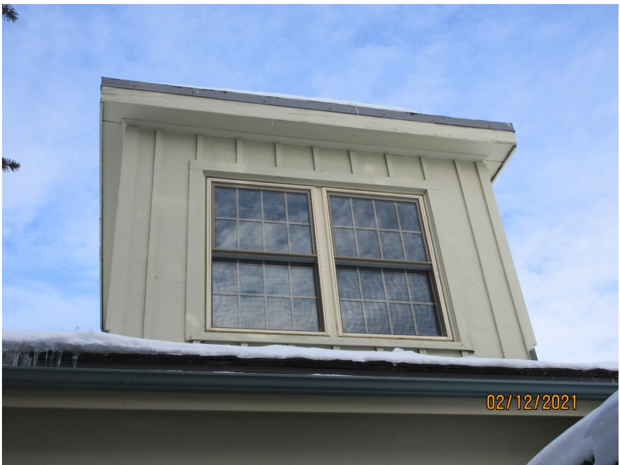
Image 28: Photograph of the shed roof dormer on the south façade of Carfrae Cottage.
