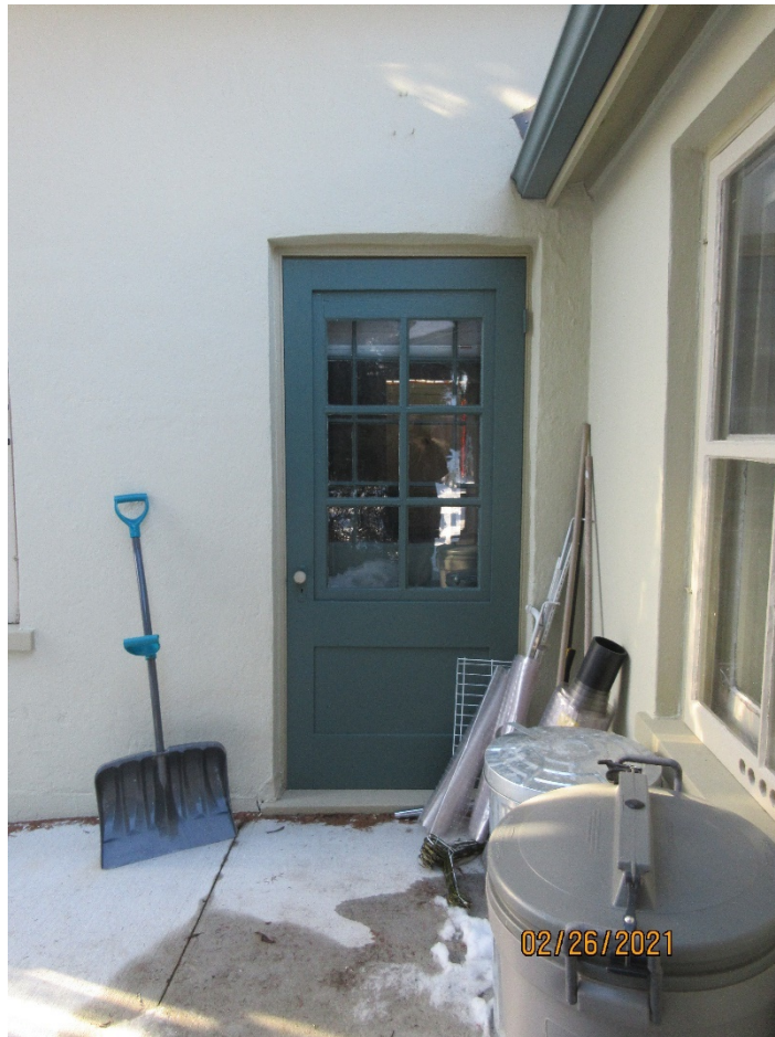
Image 24: Photograph showing the doorway, with door and storm door, on the south façade of Carfrae Cottage leading into the dining room.
