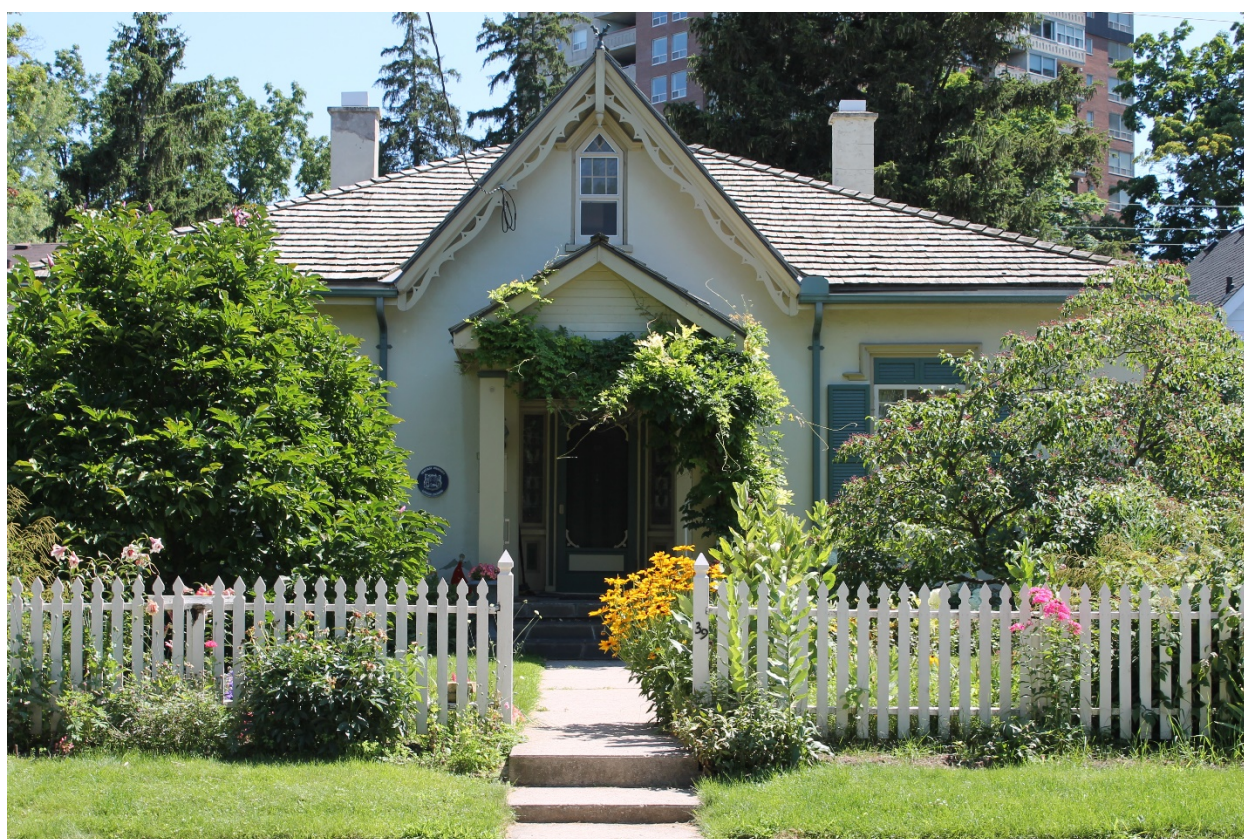
Image 2: Photograph of Carfrae Cottage on July 21, 2015.
