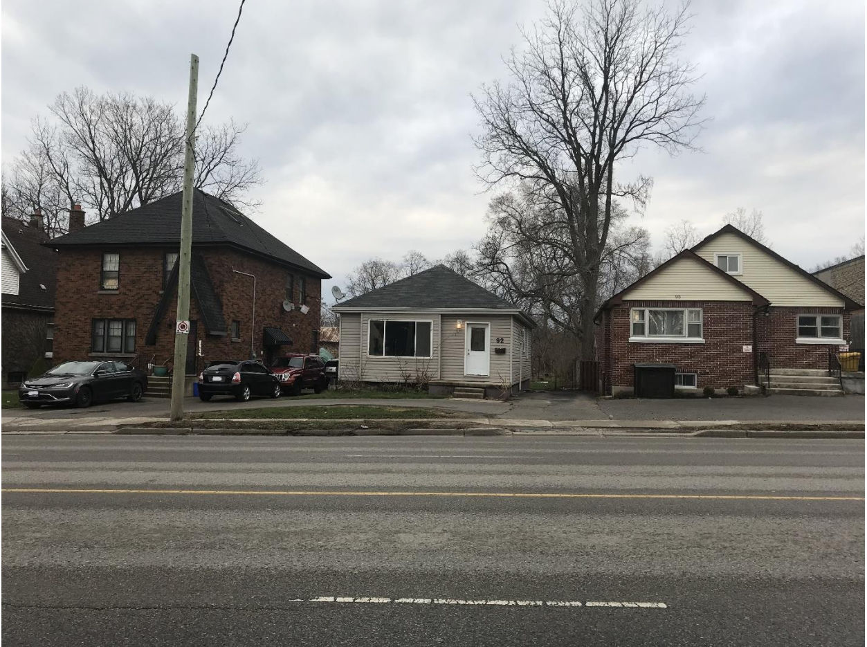
Image 1: Photograph of the subject property at 92 Wellington Road (center), seen from the west side of Wellington Road looking east (April 5, 2021).
