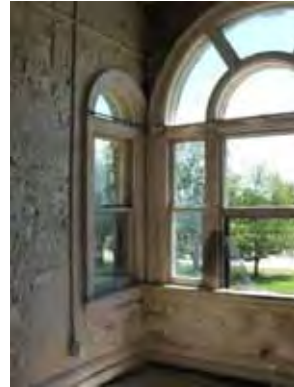
Arched window, 2 nd floor
