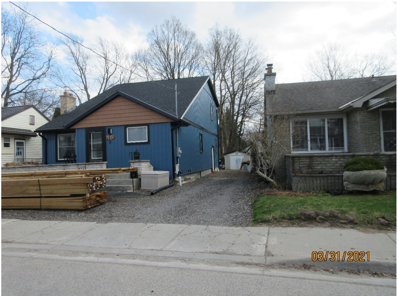
Image 8: Photograph of the subject property at 16 Cummings Avenue on March 31, 2021.
