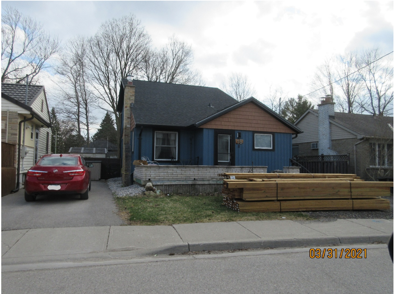
Image 7: Photograph of the subject property at 16 Cummings Avenue on March 31, 2021.
