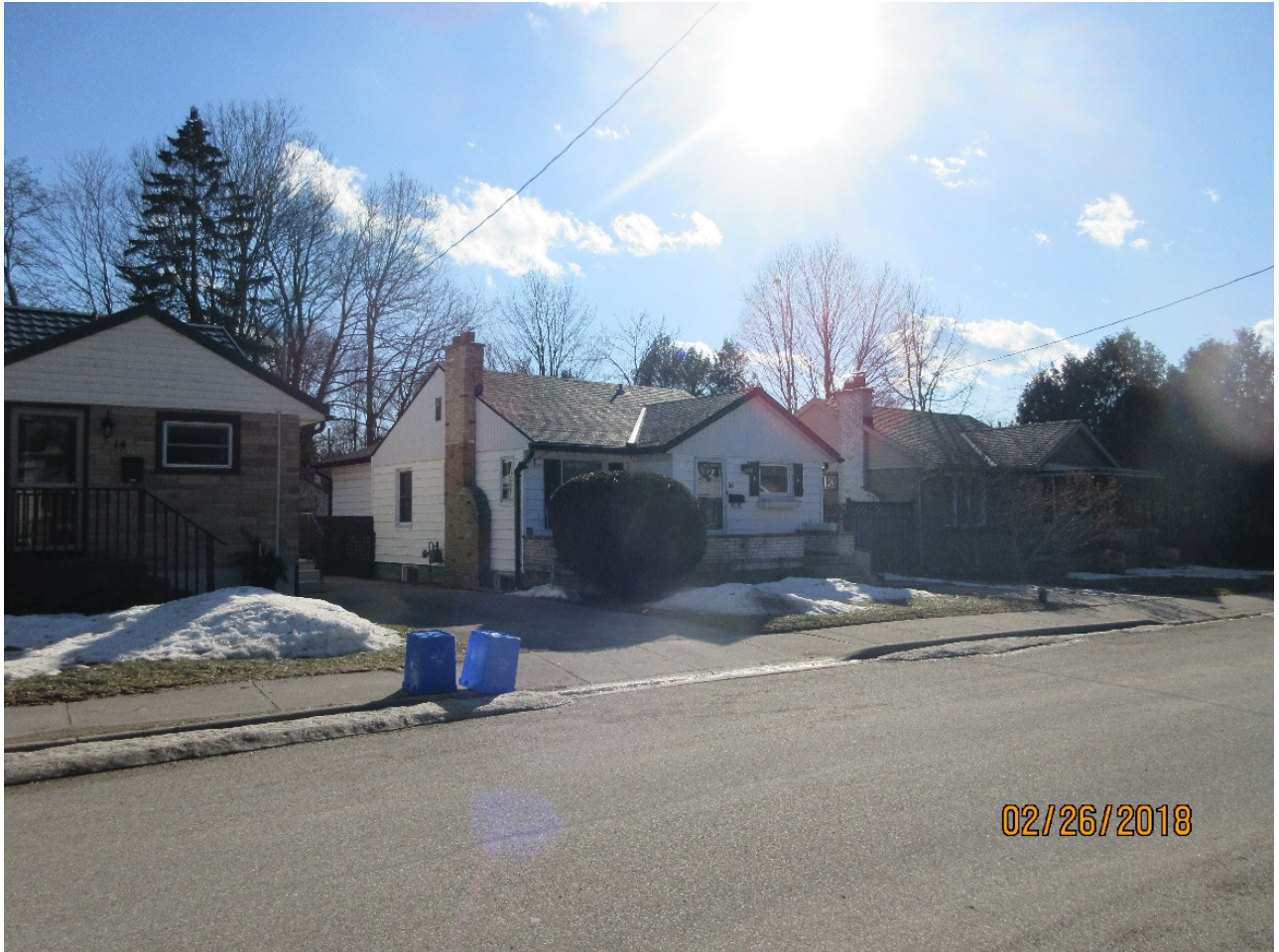
Image 3: View southwest showing the Contributing Resource at 16 Cummings Avenue prior to alterations on February 26, 2018.
