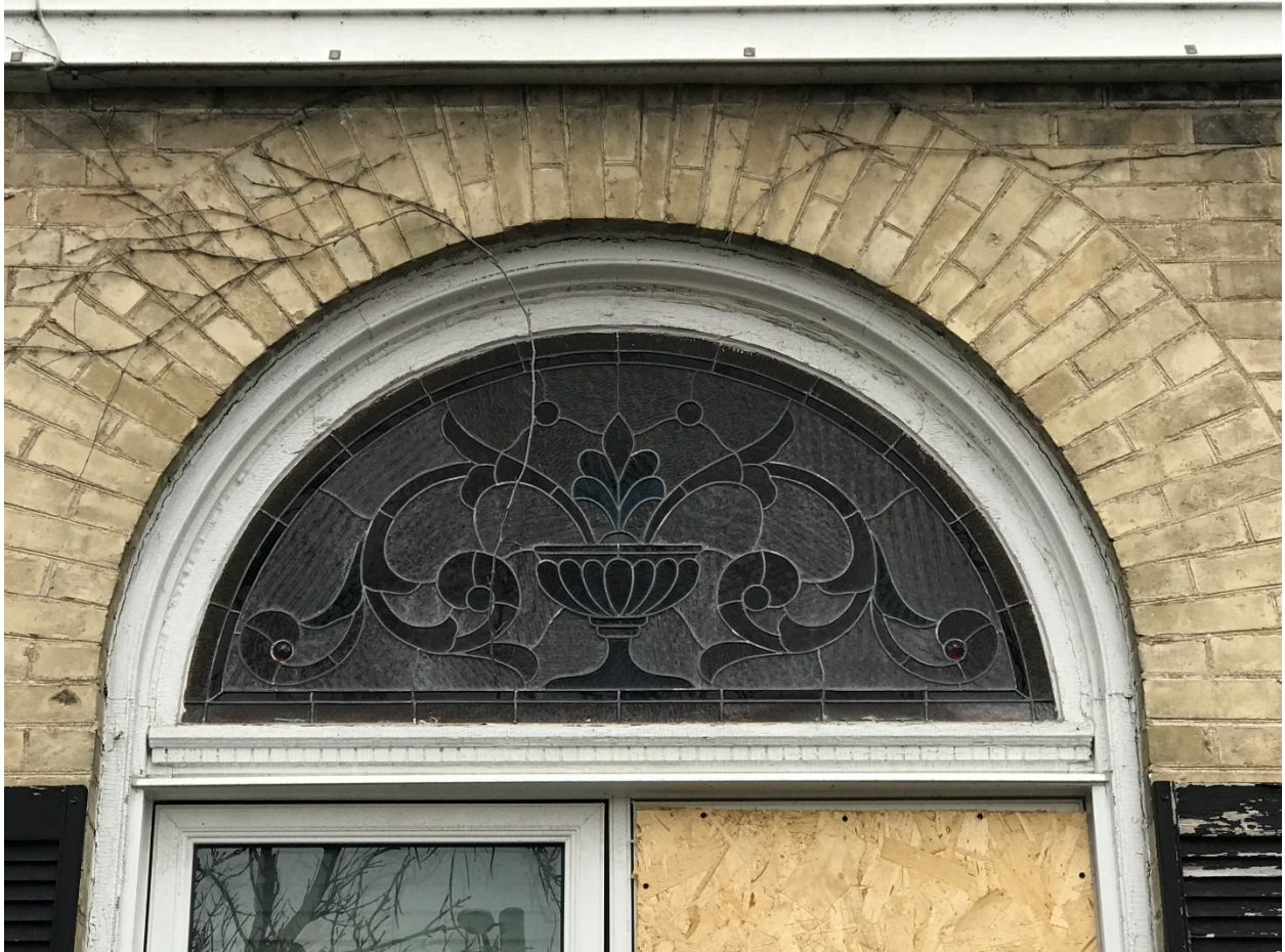
Image 3: Detail photograph of the arched transom over the front window with stained glass (April 5, 2021). The stained glass has an urn and floral motif, typical of the period of construction for the subject property. Salvage of this window in advance of demolish is strongly encouraged.
