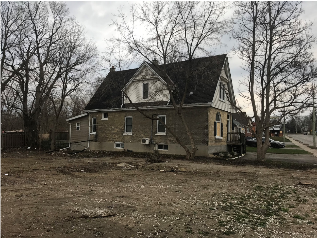
Image 2: Photograph showing the north and west (main) elevations of the building at 88 Wellington Road (April 5, 2021).
