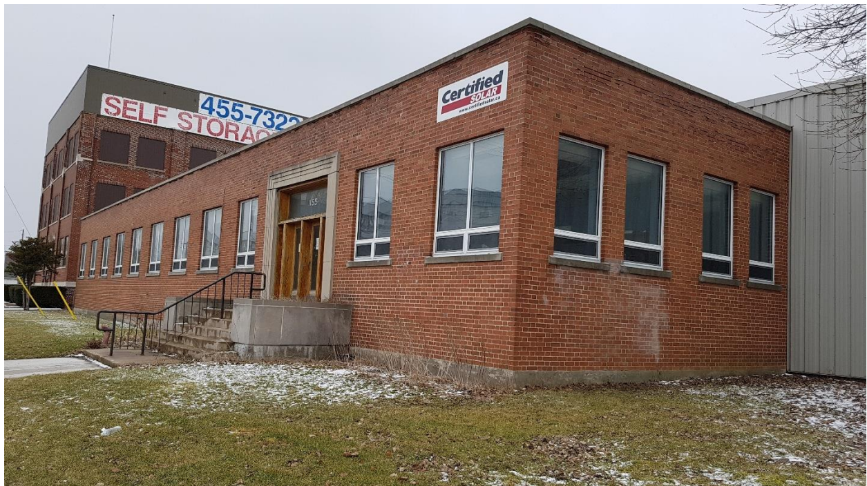
Figure 1: Front of 1153-1155 Dundas Street (facing Dundas Street)
