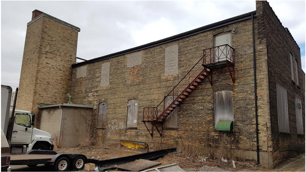
Figure 2: Rear of 1153-1155 Dundas Street (from parking lot facing King Street)
