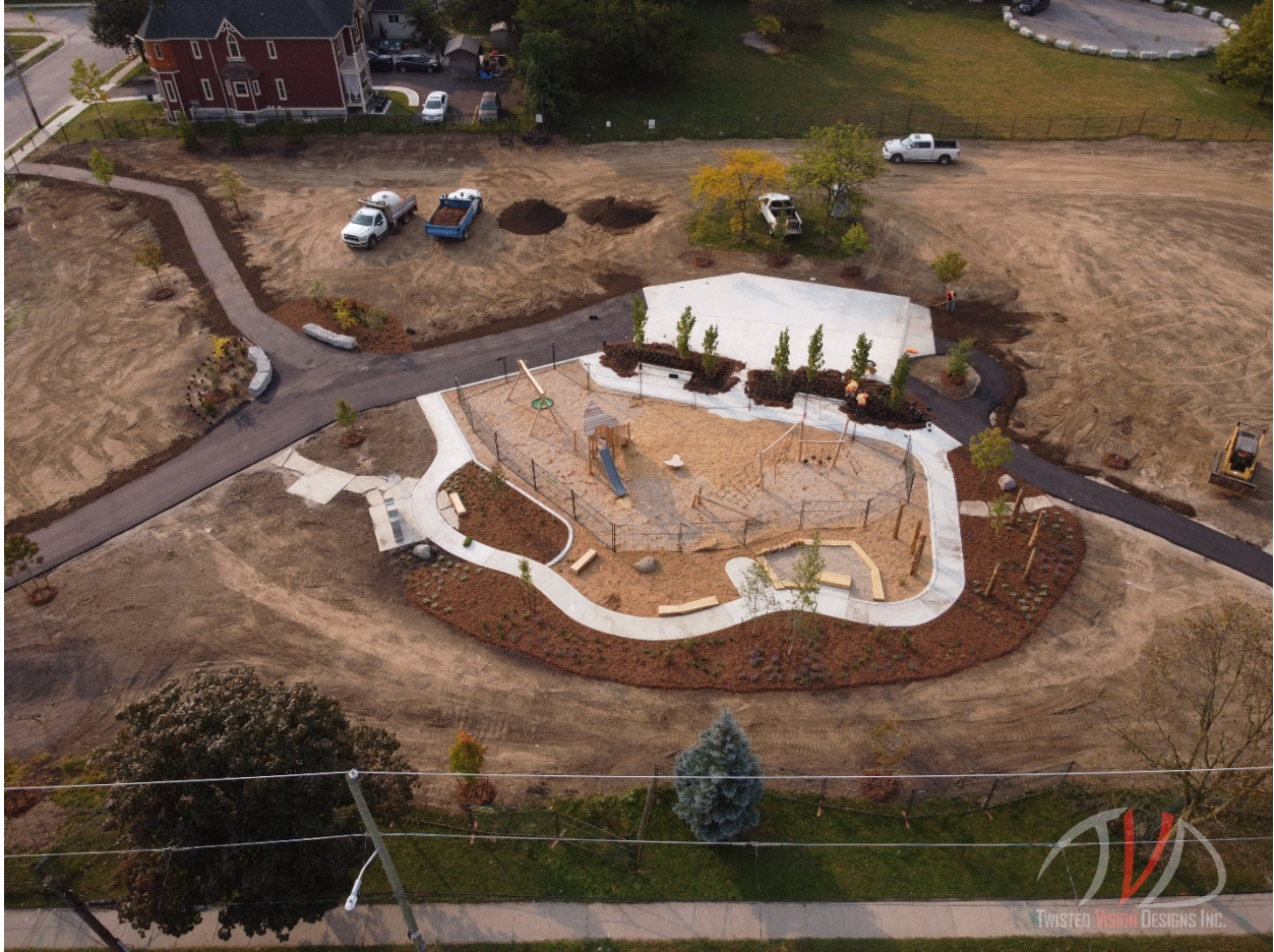
Lorne Avenue Park Playground with sensory garden (in construction)
