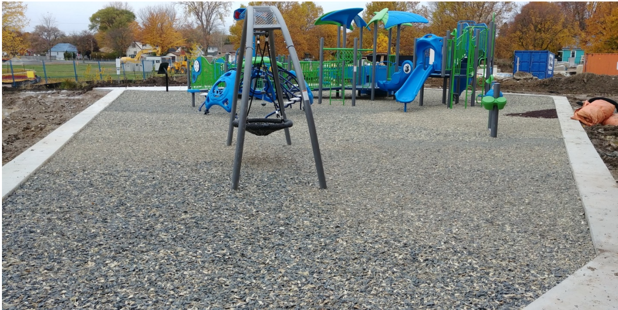
East Community Center Playground with rubber safety surfacing (in construction)
