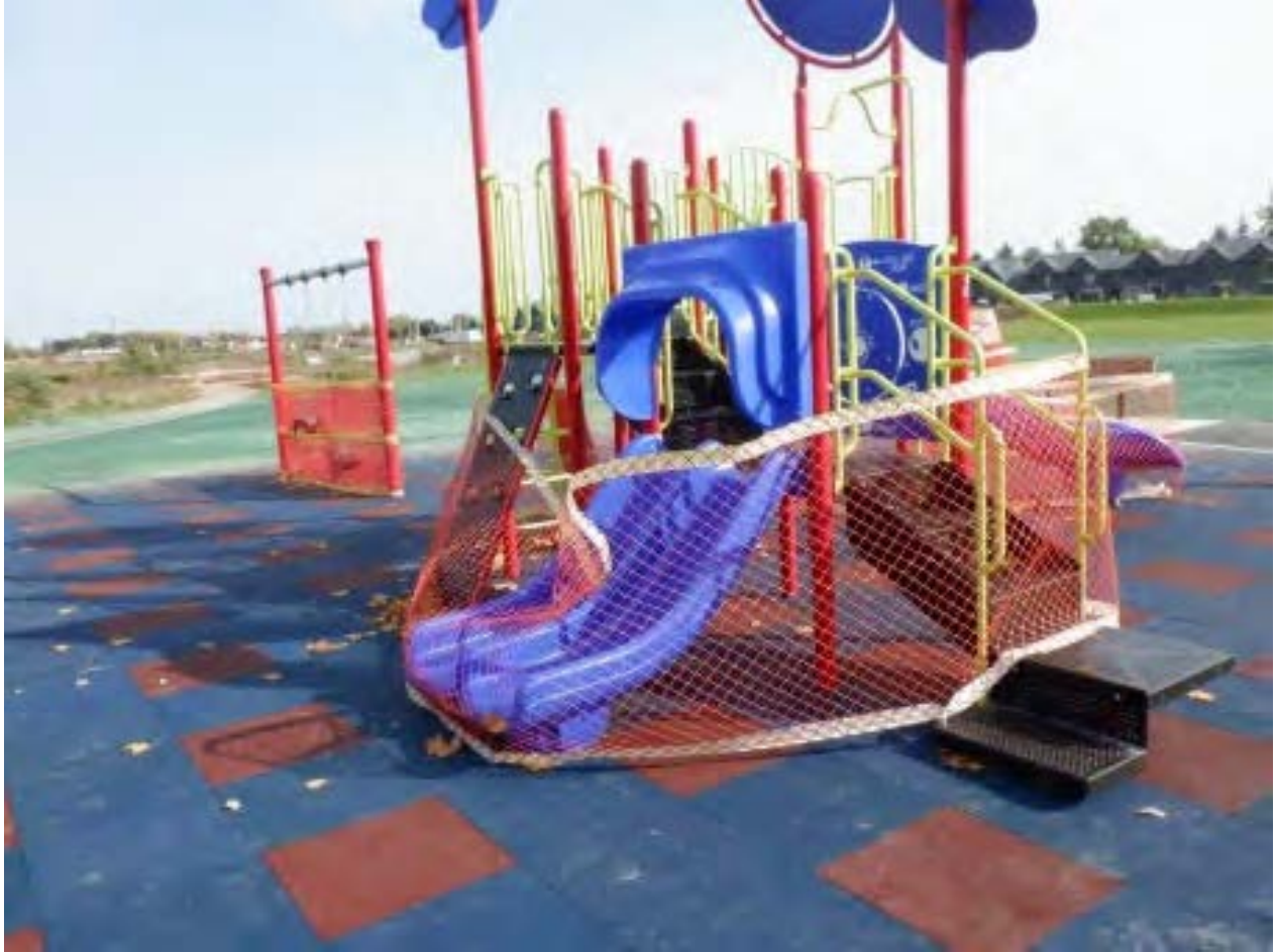
Pilot project – rubber tiles in Blackwell Park Playground (in construction)
