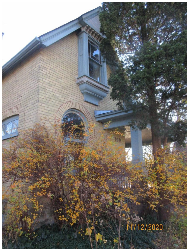
Figure 1: Exterior view of heritage dwelling located at 100 Stanley Street (November 12, 2020)
