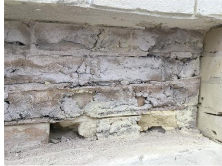
Test Cut showing Mortar between Wythes
