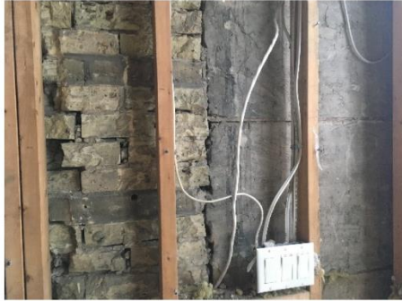
Interior Face of Masonry Wall
