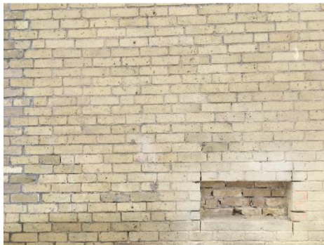
Exterior View of East Wall and Test Cut
