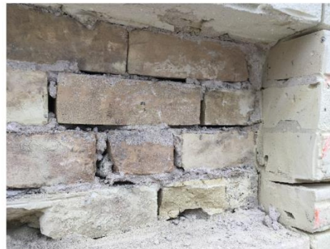
Test Cut showing Interior Brick Wythe
