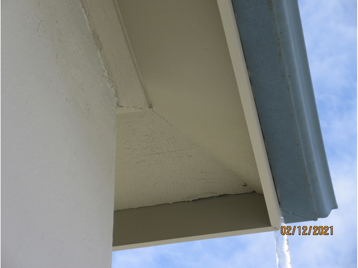
Image 10: Photograph showing the sloped, painted wood soffit of the roofline.
