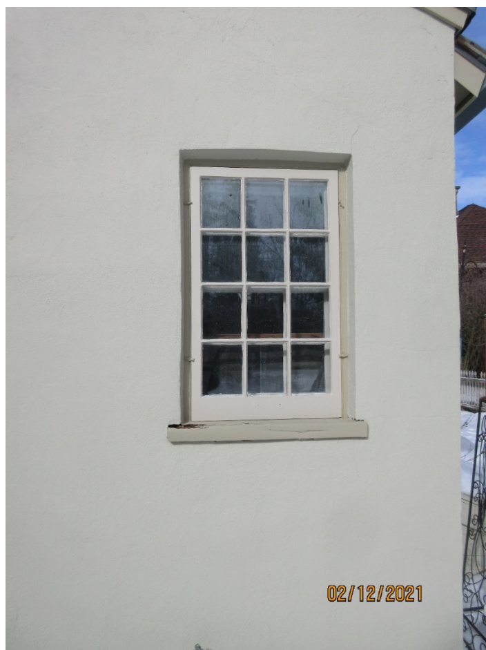
Image 29: Photograph of the six-over-six painted wood window on the south façade of the kitchen wing with a matching wood storm window and wood sill.
