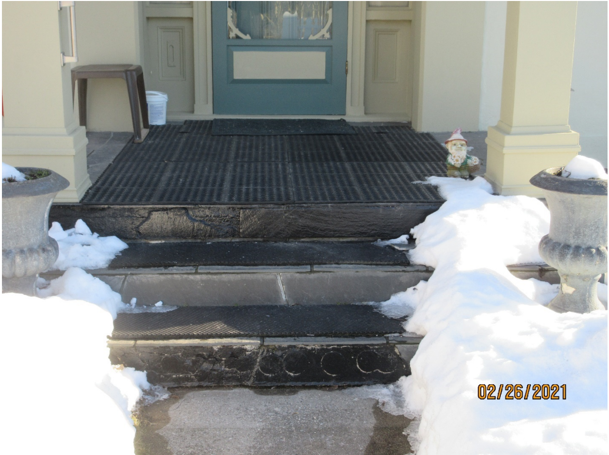
Image 15: Photograph showing the existing condition of the porch base.
