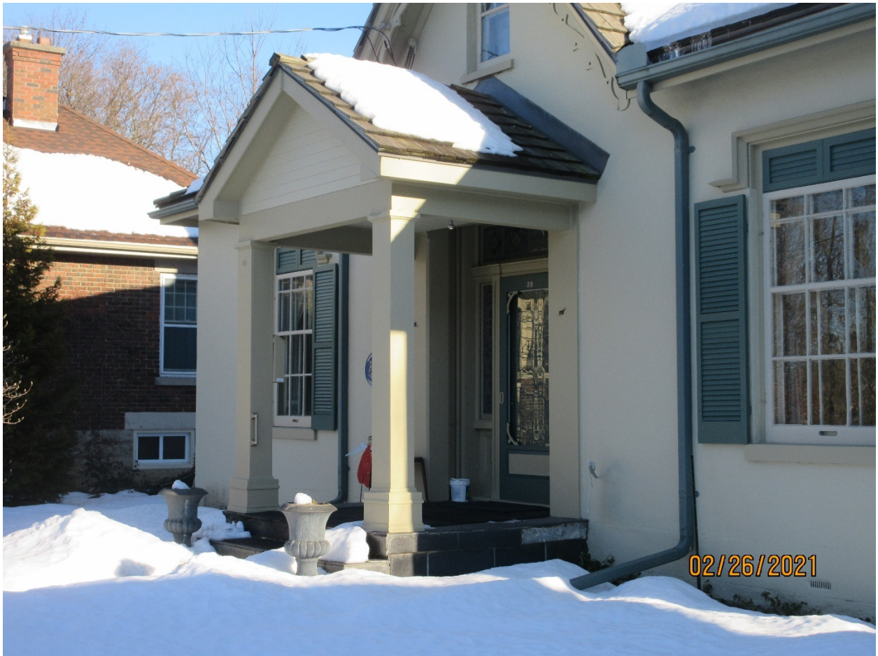
Image 14: Photograph showing the simple form of the painted wood porch over the front doorway, which fails to detract from the original structure, with a cedar shingle gable roof, supported by a plain frieze and boxed piers with simple capital and base details.
