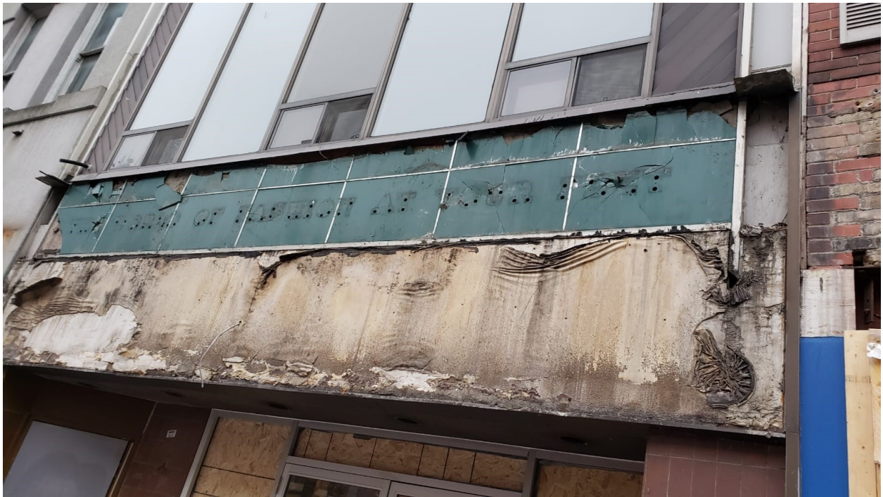
Image 4: Detail of the materials located behind the previously installed sign-box. The ghosting left on what appears to be vitrolite states "THE WORLD OF FASHION AT YOUR FEET" likely associated with one of the mid-20th century shoe retailers that occupied the storefront.
