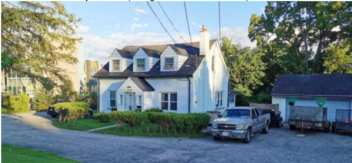
Figure 1. Front view of the subject lands (facing south on Sarnia Road)
