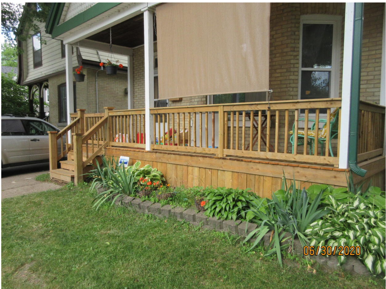
Image 4: Detail of the porch at 61 Wilson Avenue.
