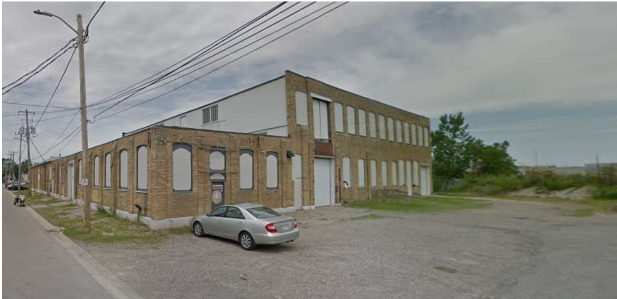
Photo 1 – Existing Building at 820 Cabell Street (Source: Google Streetview)
