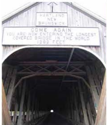
The Hartland Covered Bridge crossing the St. John River at Hartland, NB, is the world's longest covered bridge. It is significant for its structural qualities, contributions to transportation and as a symbol of the heritage of covered bridges in New Brunswick. The present bridge is a standard covered bridge structure composed of a Howe truss superstructure enclosed with vertical unpainted weatherboard siding. When the New Brunswick Department of Transportation recently rehabilitated the bridge by installing a fire suppression system, care was taken to ensure that this new system was barely visible in the upper structural system.
