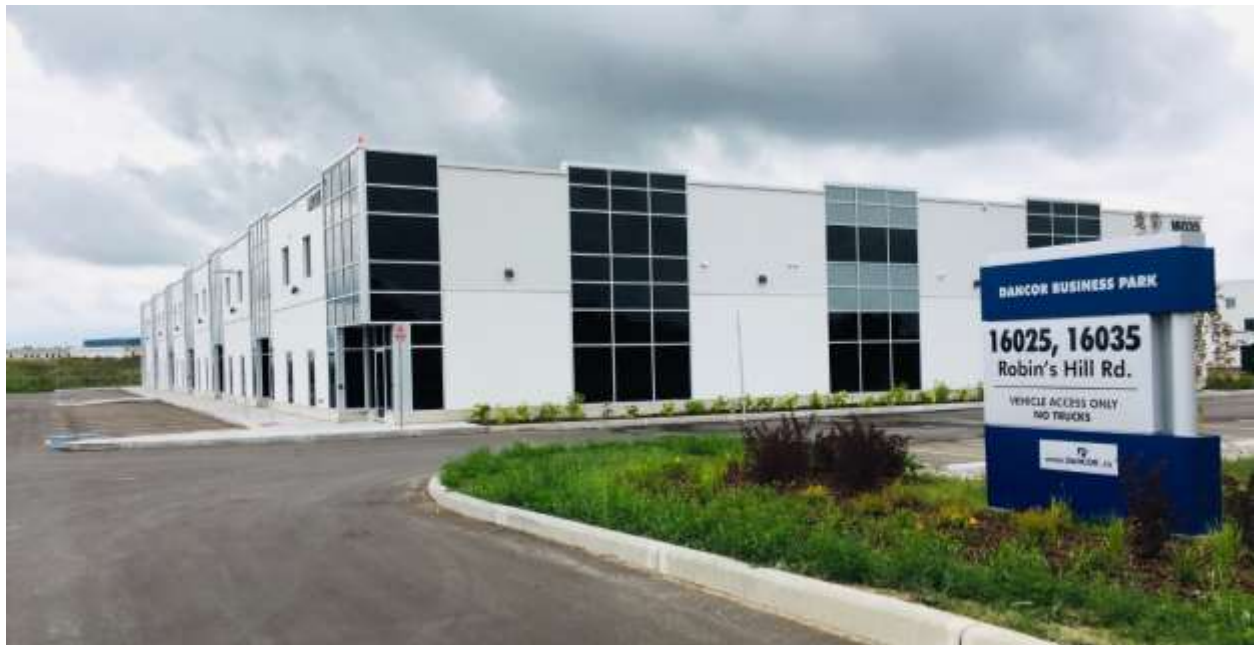
Figure 1. Building at 16035 Robin's Hill Road
