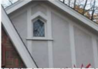
1. Half-timbering set in textured stucco
