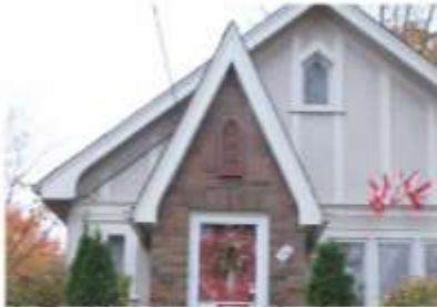
4. Red brickwork with alternating darker brick set randomly, with a soldier course and a basket weave bond over the front doorway
