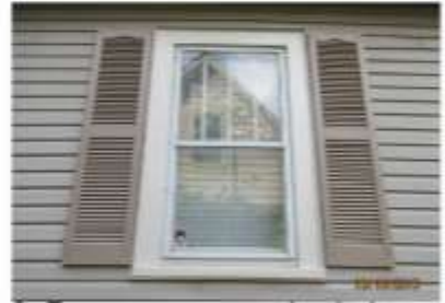
9. Four-over-one sash window at rear, originally the Curnoe boys' bedroom window, portrayed in Greg Curnoe's 1972 painting, Backyard, Langarth St. E.
