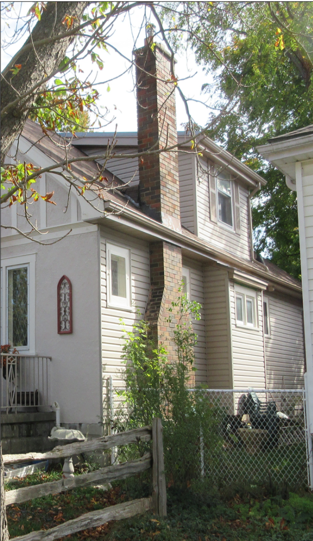
Red brick chimney flanked by pair of leaded windows, dormer and projecting oriel window from dining-room on west elevation—Photo: Kyle Gonyou
