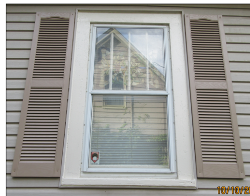
4-over-1 windows; storm windows added by Stan Porter—Photo: Kyle Gonyou
