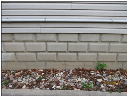
Concrete block foundation to look like dressed stone—Photo: Kyle Gonyou
