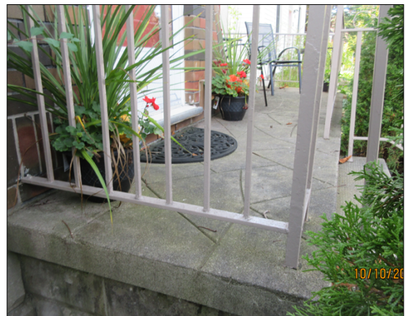
Porch railing and stamped concrete porch floor Photo: Kyle Gonyou
