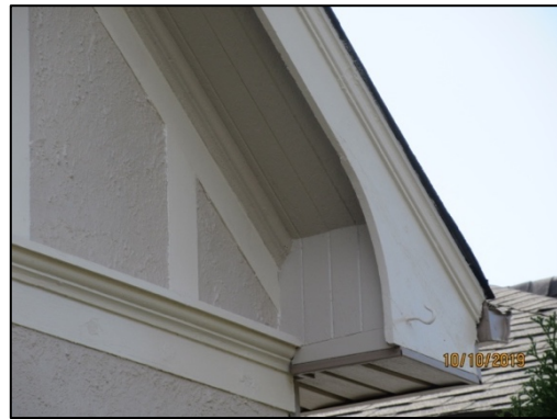
Wood soffits, moulded bargeboard with prominent gable ends—Photo: Kyle Gonyou
