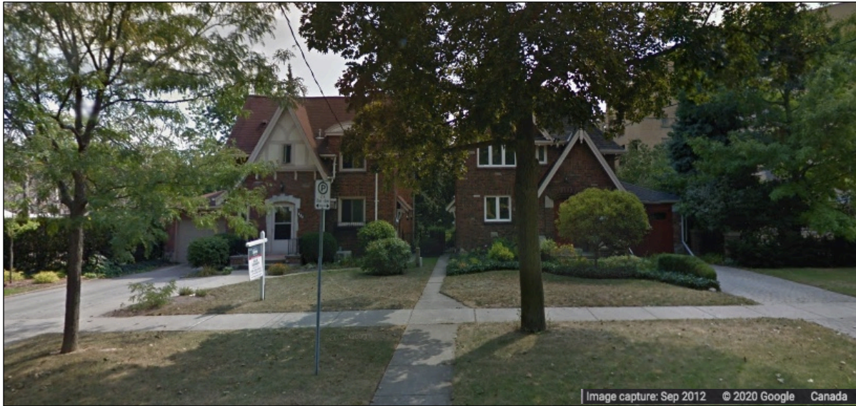
253 St James Street (left) and 251 St James Street (right) Part V Designation: Bishop Hellmuth Heritage Conservation District
