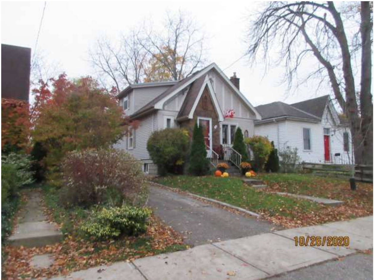
Image 3: View of the property at 75 Langarth Street East showing the front (north) and east facades.
