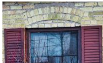
11. The single-storey wash house to the west side also exhibits a segmental-arch window with brick voussoir
