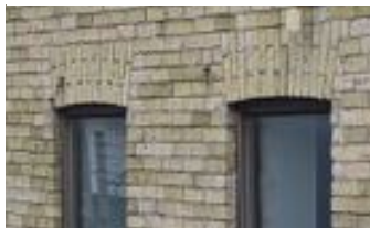
10. Most of the original windows are segmental arch openings topped with brick voussoirs
