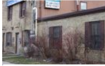
2. And to its function as a vernacular mid-19th century proto-industrial structure
