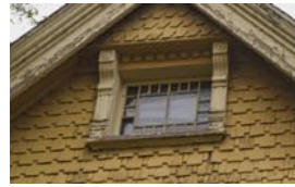
9. There is a small square gable window under the eaves. There is a pilaster on each side of the window frame. The window is divided in two and surrounded by a border of small square panes
