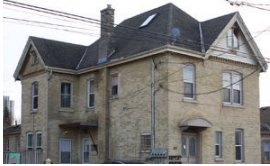
4. The roof is irregular with a shallow gabled profile. It has a cross gable and two gable ends
