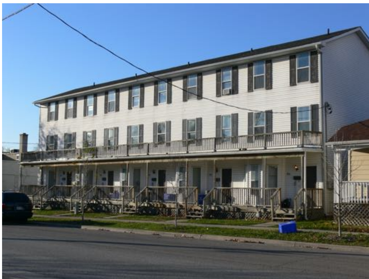
The row-houses at 146-154 Ann Street
