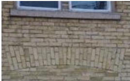
11. On the second storey of the front façade are double windows, which were apparently echoed on the first storey
