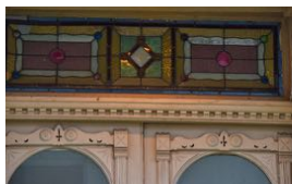
17. The doorway has a dentil-moulded architrave above
