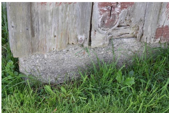
Plate 23: Concrete foundation, looking south
