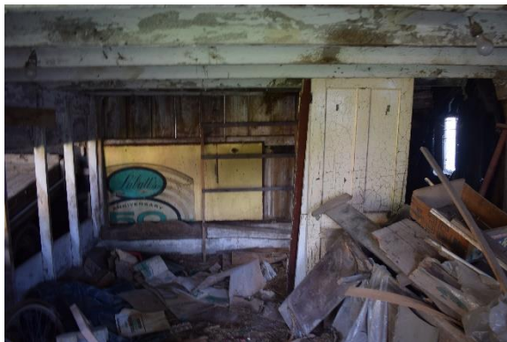
Plate 36: Storage area, looking north
