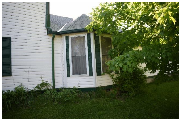
Plate 17: Bay window, looking east
