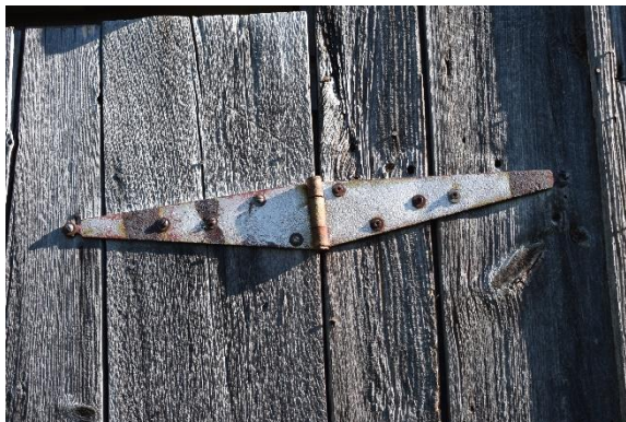
Plate 30: Metal hinge on door, looking north
