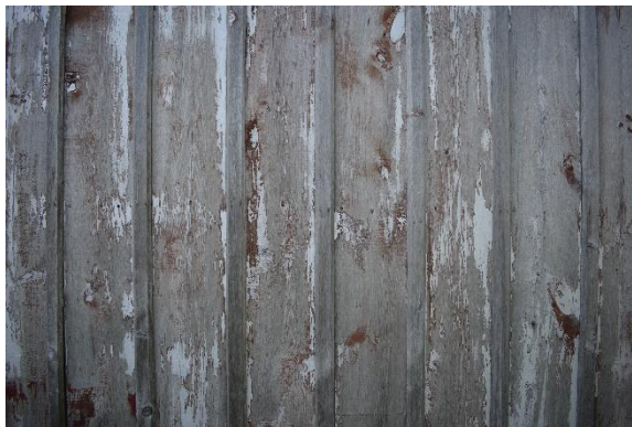
Plate 22: Board and batten siding, looking south
