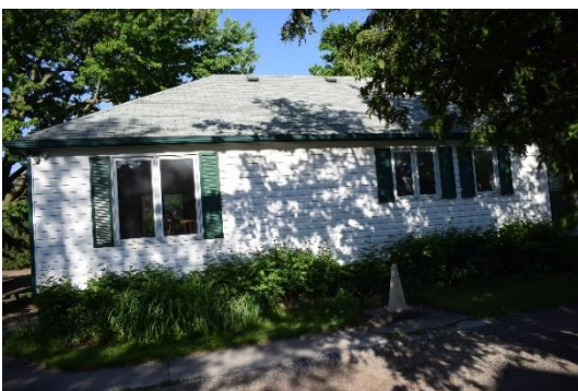
Plate 15: East façade of the addition, looking west
