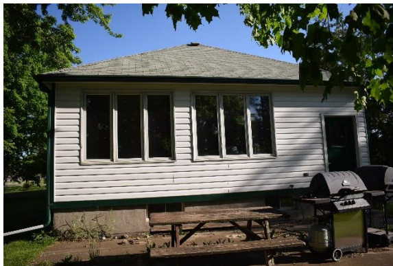
Plate 20: South façade, looking north
