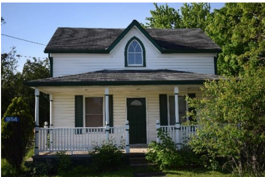
Plate 11: Front façade of residence, looking south
