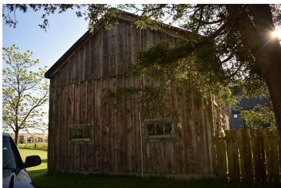
Plate 27: West façade, looking east
