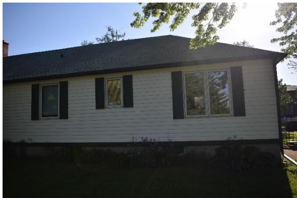
Plate 19: West façade of modern addition, looking east
