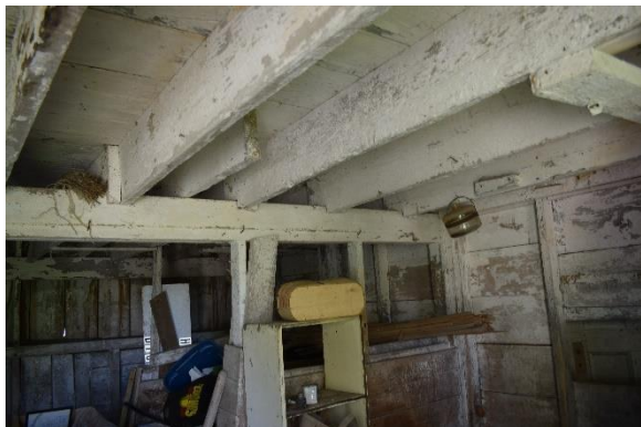
Plate 33: Joists and beams, looking north
