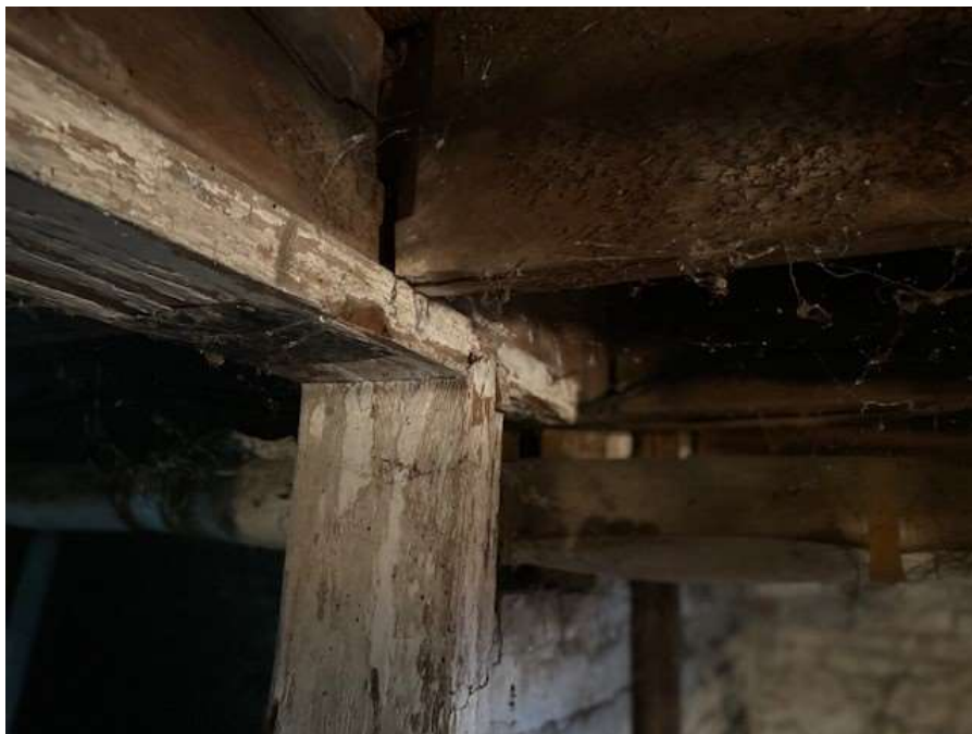
Image 14: Basement of original farmhouse showing post and floor joist detail
