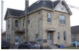
2. However, this is a larger and more imposing structure than a typical Queen Anne cottage
