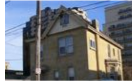
3. The house is built of buff London brick. The house has the typical irregular and stepped outline and profile of this style
