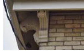
5. There are brackets below the roof at the principal corners
