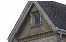
7. The gable ends exhibit wood shingling. The front façade gable is clad with siding but the east gable exhibits the original bargeboard shingling and is outlined with moulded vergeboards
