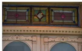
17. The doorway has a dentil-moulded architrave above
