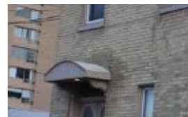
18. The porch roof of the doorway is altered but appears to adhere to the line of a previous porch and is still supported by original brackets
