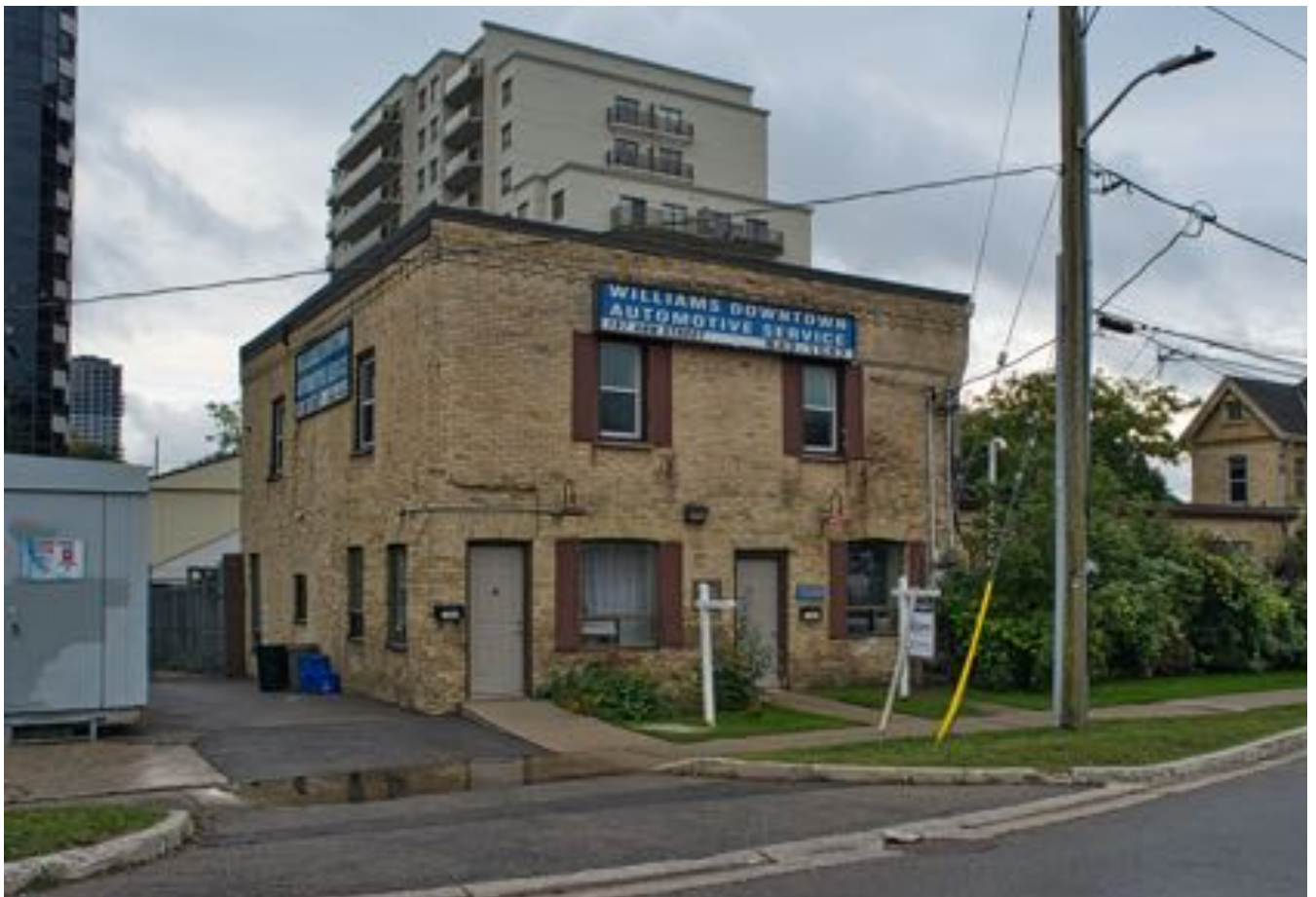
Kent Brewery building, October 2020
