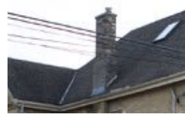
6. There are two buff brick chimneys
