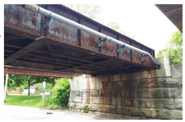
**Property Description:** This property consists of an iron through-girder railway bridge with wood railway ties, rails overhead, and a foundation of coursed ashlar masonry blocks. It is located south of the intersection of Oxford Street East and Talbot Street, and Talbot Street passes underneath the bridge.
