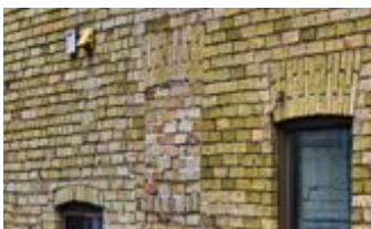
13. Though largely preserving the original sills and voussoirs
