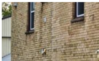
16. A line of demarcation in the brick is apparent in the middle of the east side of the building showing alterations
