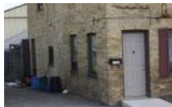
9. The extant front door is to the side of the frontage, breaking the usual symmetry of the Georgian style and pointing up its utilitarian function where floor space is needed inside for production
