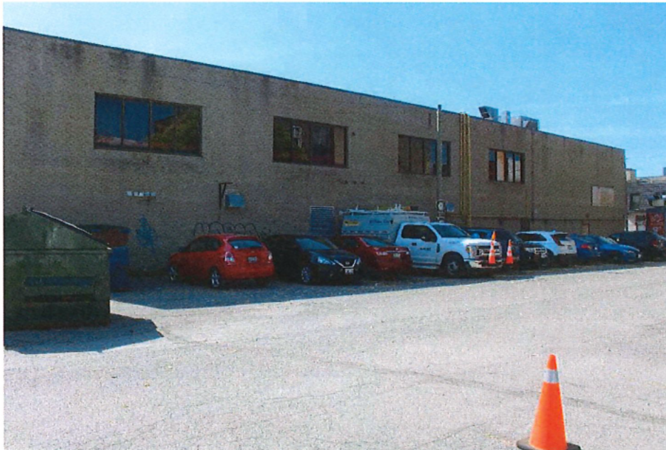
Image 10: View showing 120 York Street from the south, September 2019
