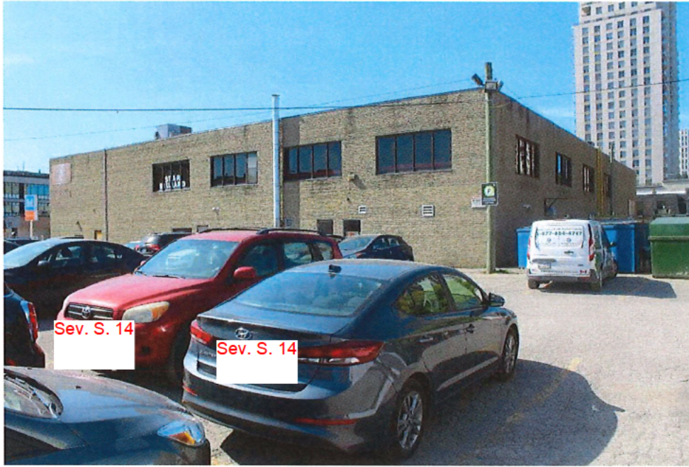
Image 9: View showing 120 York Street from the east, September 2019
