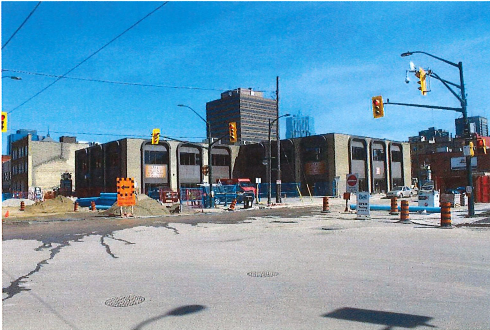
Image 5: View showing 120 York Street from the south, September 2019
