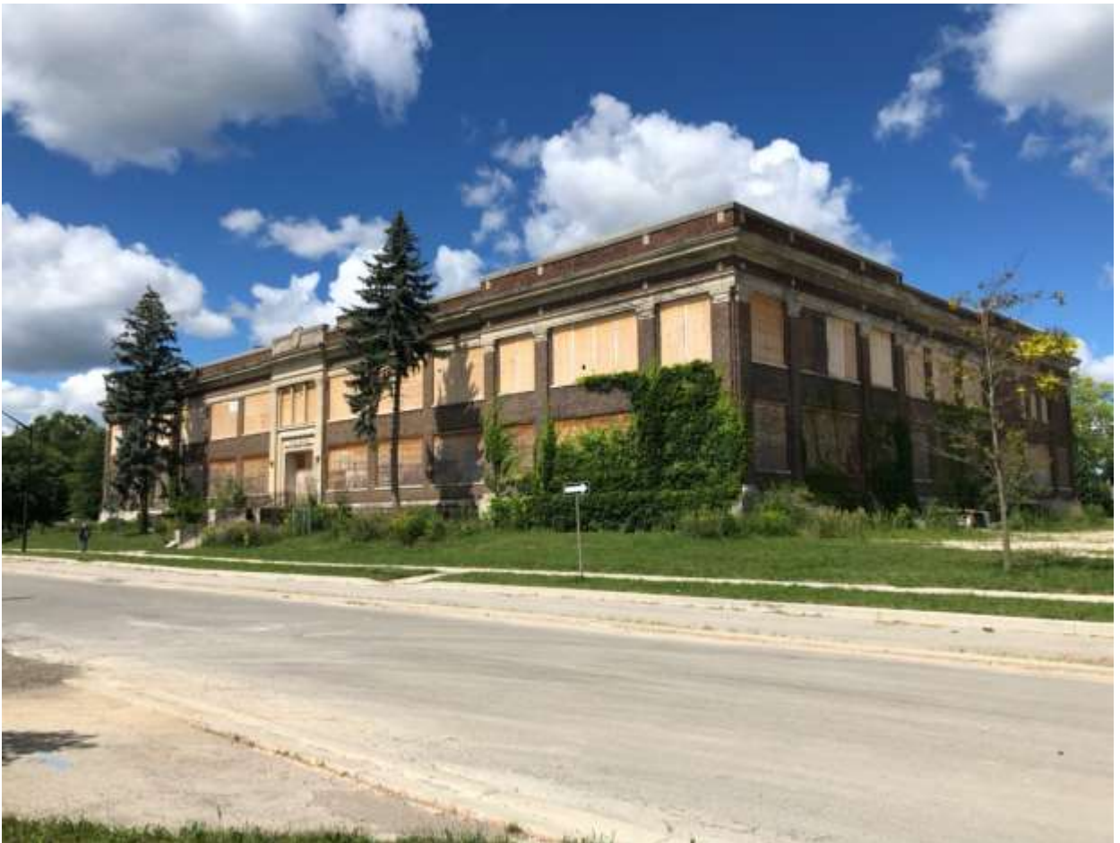
Figure 2: Health Sciences Building (northwest view from South Street)
