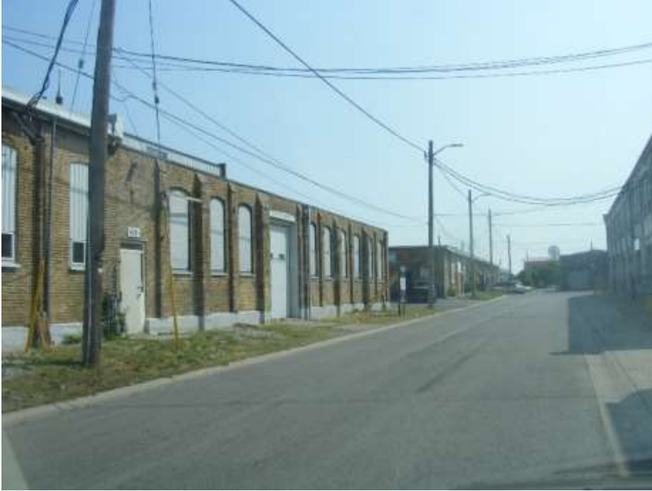
Photo 3 – Door on Cabell Street
