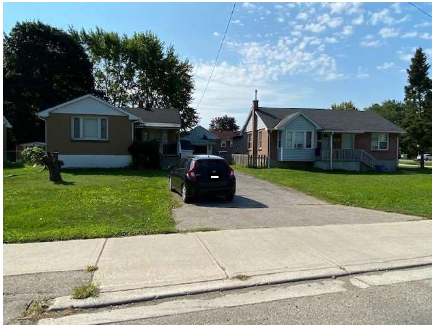
Image 5: 1455 and adjacent property at 1453 Oxford Street – street elevations (August 24, 2020)
