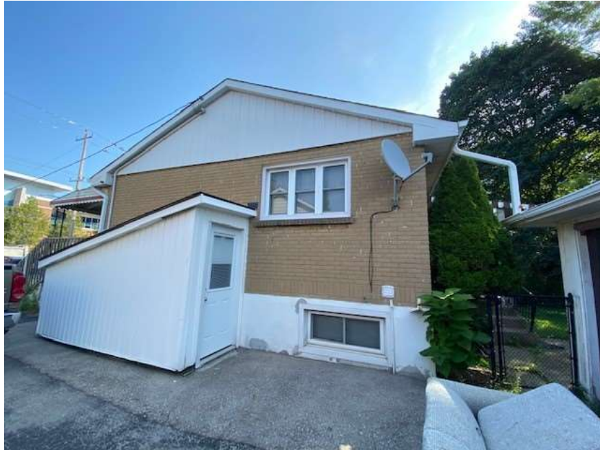
Image 4: 1455 Oxford Street East – view of east-side elevation (August 24, 2020)
