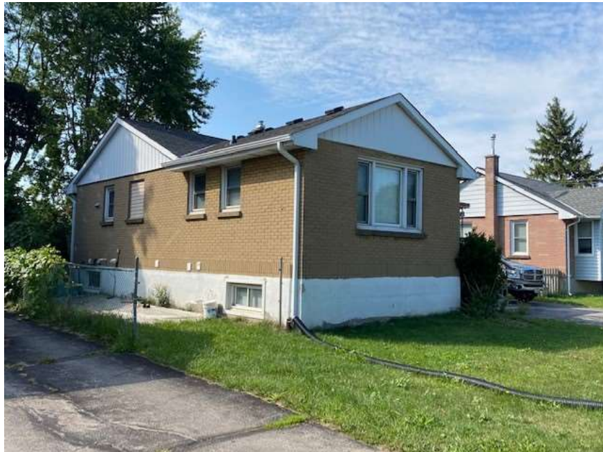
Image 2: 1455 Oxford Street East – view of corner, front and east-side elevations (August 24, 2020)
