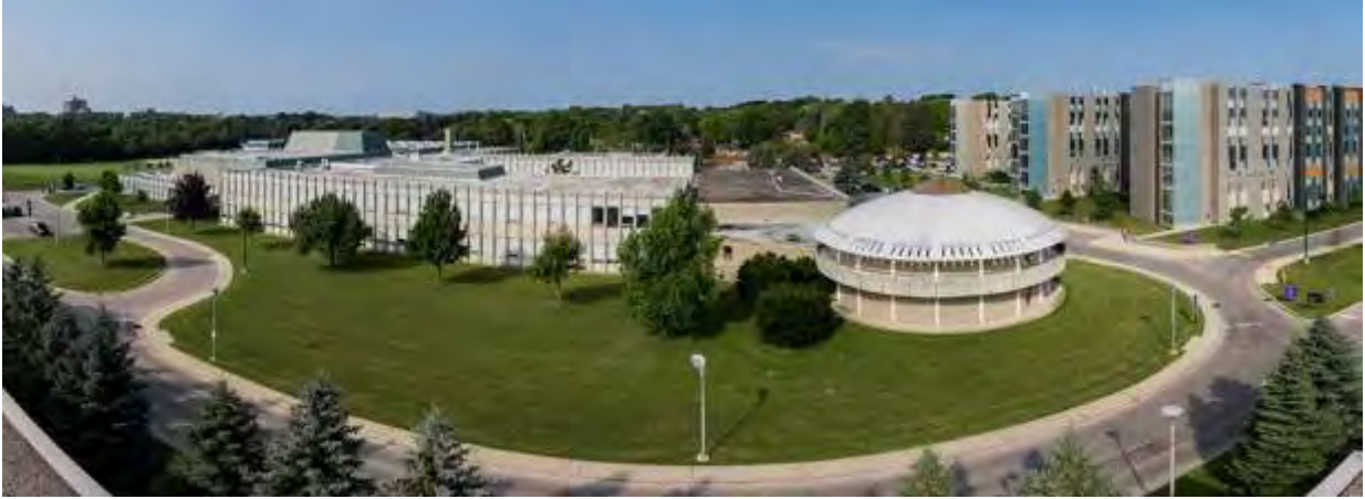
Figure 8: Birds eye view of the John G. Althouse building, looking north-west (Source: Western University (website), accessed 2020)
