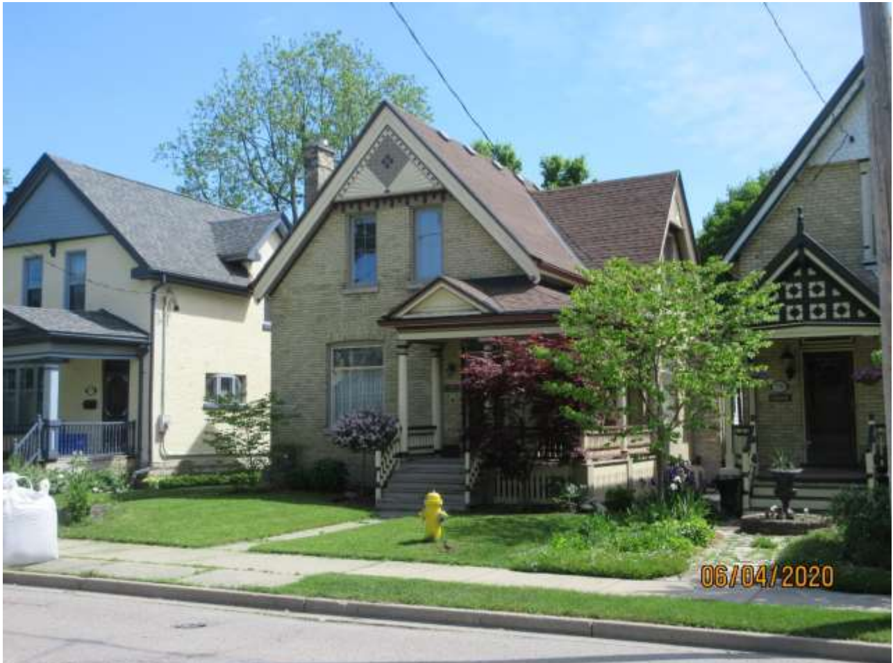
Image 3: Photograph showing the property at 784 Hellmuth Avenue following the replacement of the windows without Heritage Alteration Permit approval.
