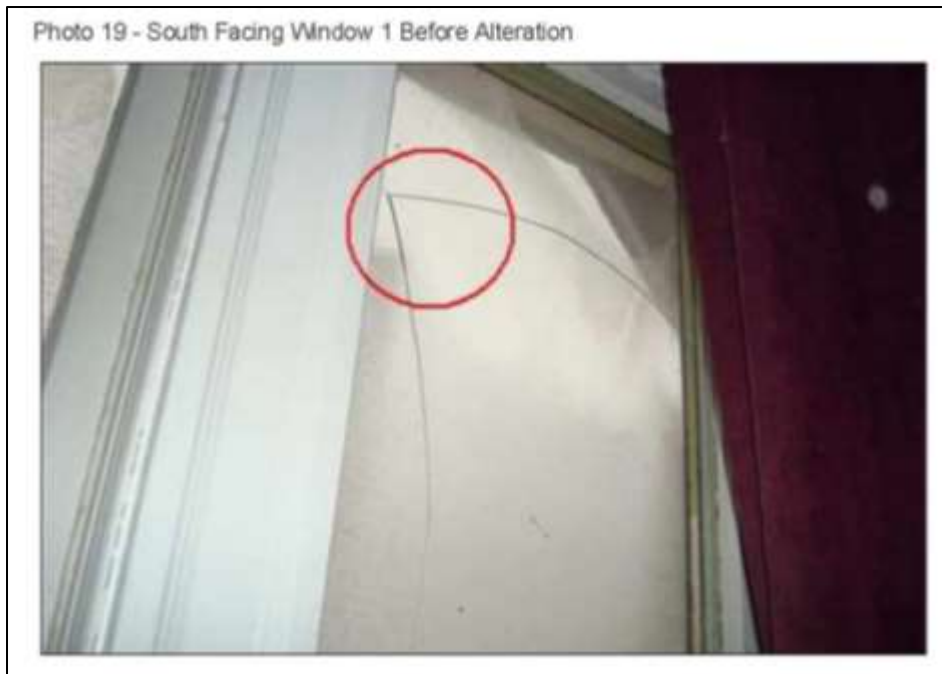
Image 11: Image of the south facing window 1 before alteration (interior), submitted as part of the Heritage Alteration Permit application. Circle on image identifying crack in the glass pane.
