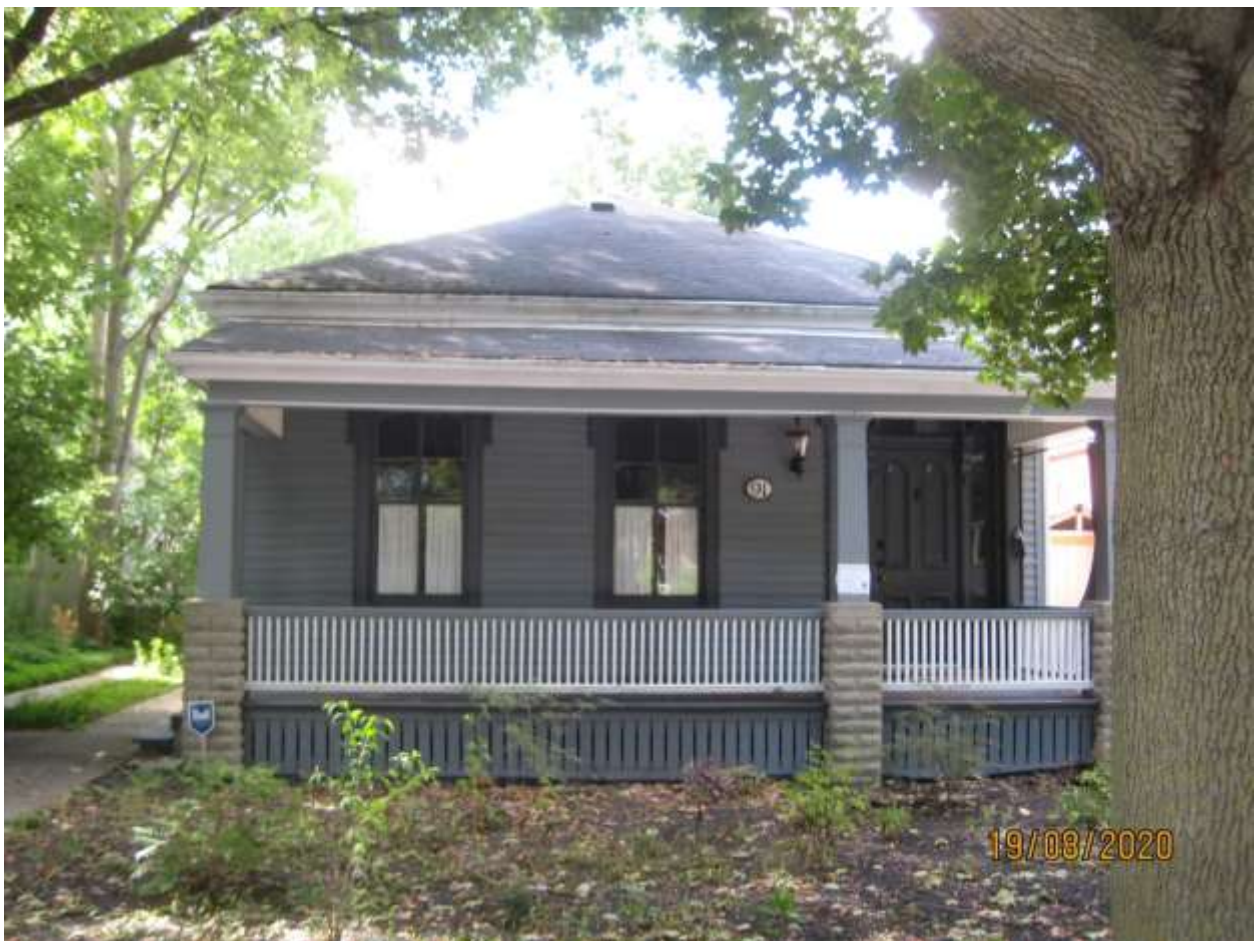
Image 4: Photograph showing the existing conditions of the dwelling at 91 Bruce Street in the Wortley Village-Old South Heritage Conservation District. Note, the railing on the right side of the photograph is proposed to be removed as a part of the proposed porch restoration.
