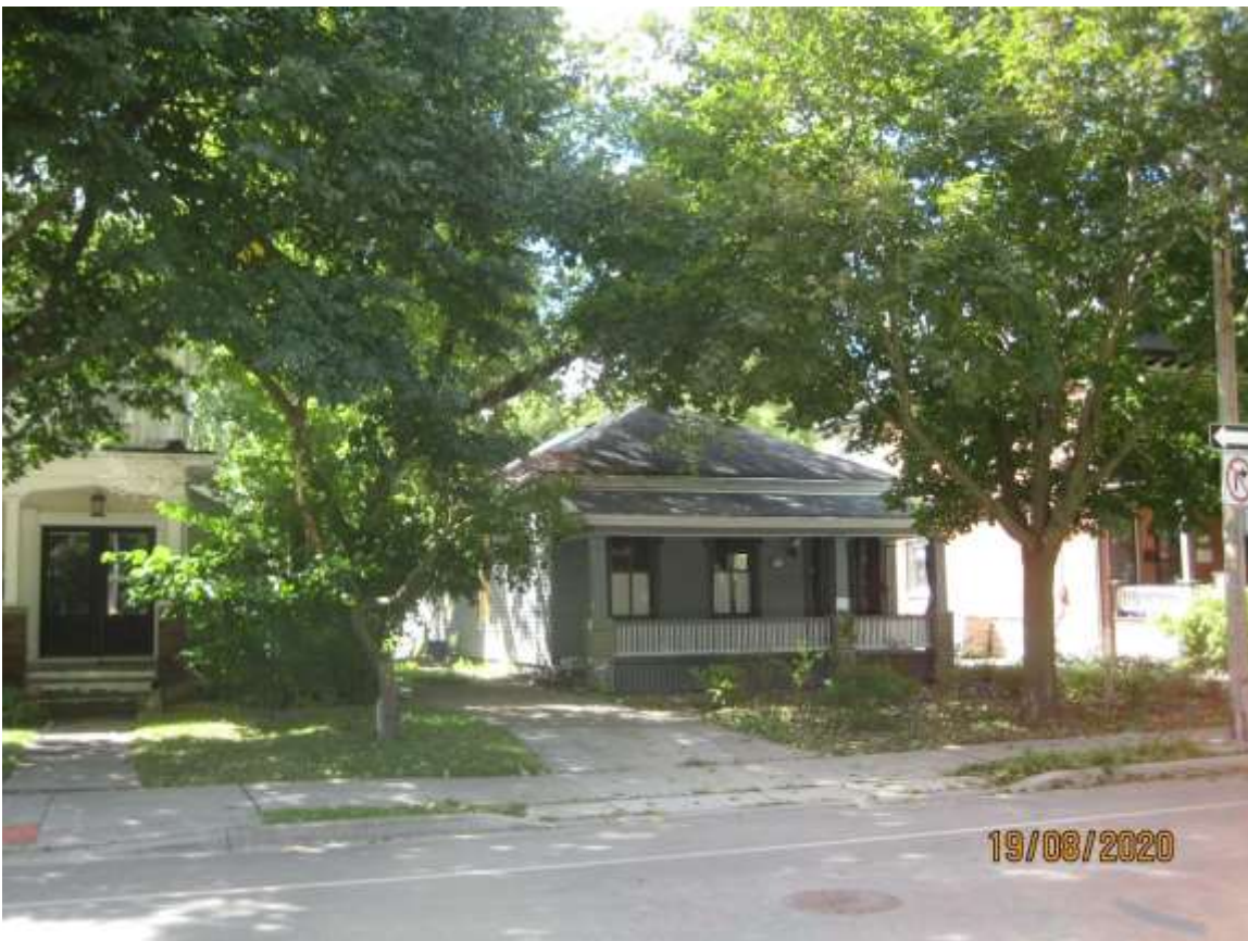
Image 6: Photograph showing the front (north) and side (east) facades of the dwelling, showing its existing conditions as view from the north side of Bruce Street.
