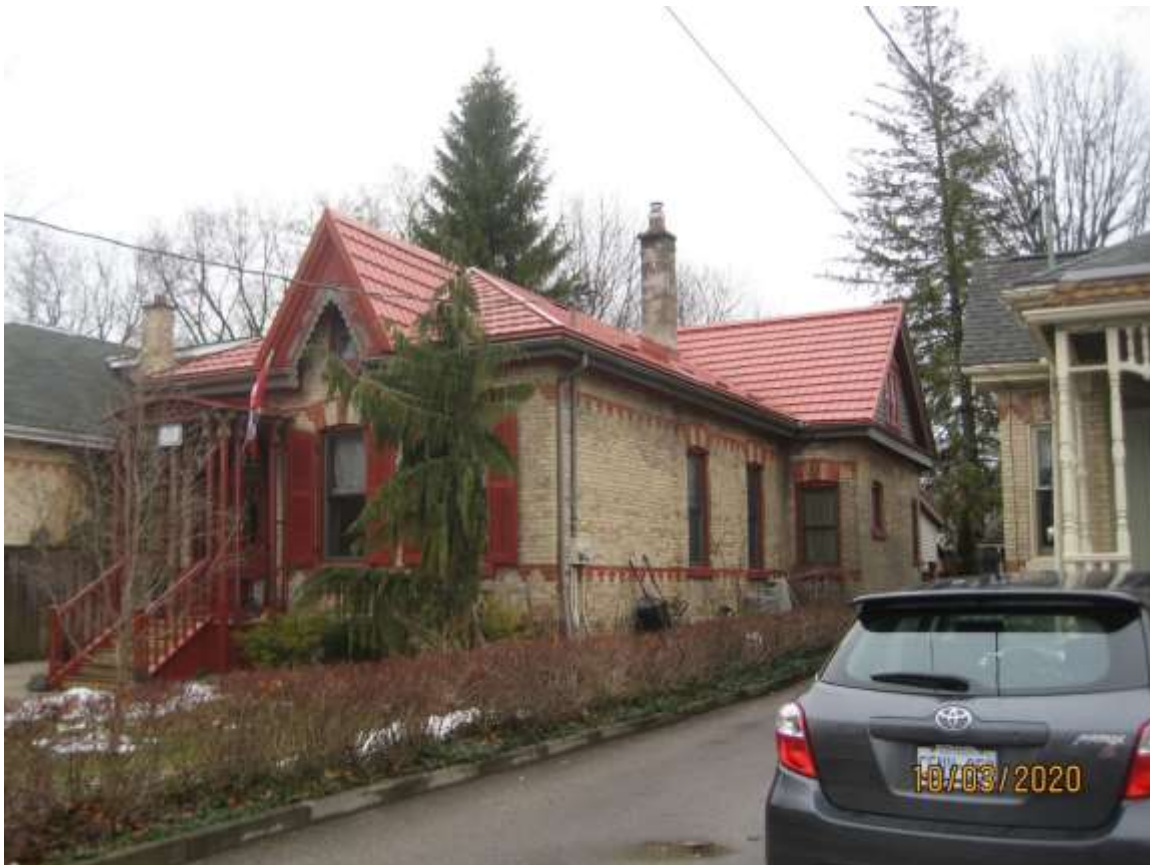
Image 10: Photograph of the property located at 43 Bruce Street, in the Wortley Village-Old South Heritage Conservation District showing a side hall plan cottage, similar in scale to the subject property. A cross gable has been previously add onto the dwelling to allow for an increased building height and addition half storey. The property was cited in the Heritage Alteration Permit application as a design importation for the cross gable proposed at 91 Bruce Street.
