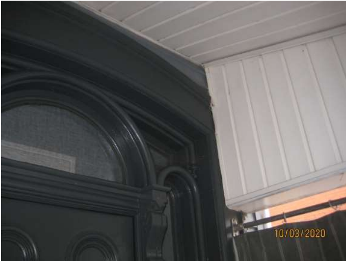
Image 9: Detail showing the existing conditions of the London Doorway. Note, the trim of the doorway has been previously altered with the installation of the porch ends. The Heritage Alteration Permit application seeks to restore the porch ends and porch ceiling in a manner that exposes the trim of the doorway and allows for the future restoration of the London Doorway.
